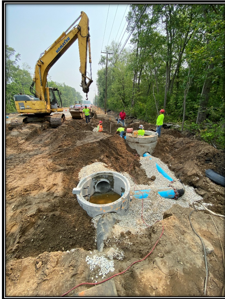
Figure: P&A Construction installing the dual vortex separators.
