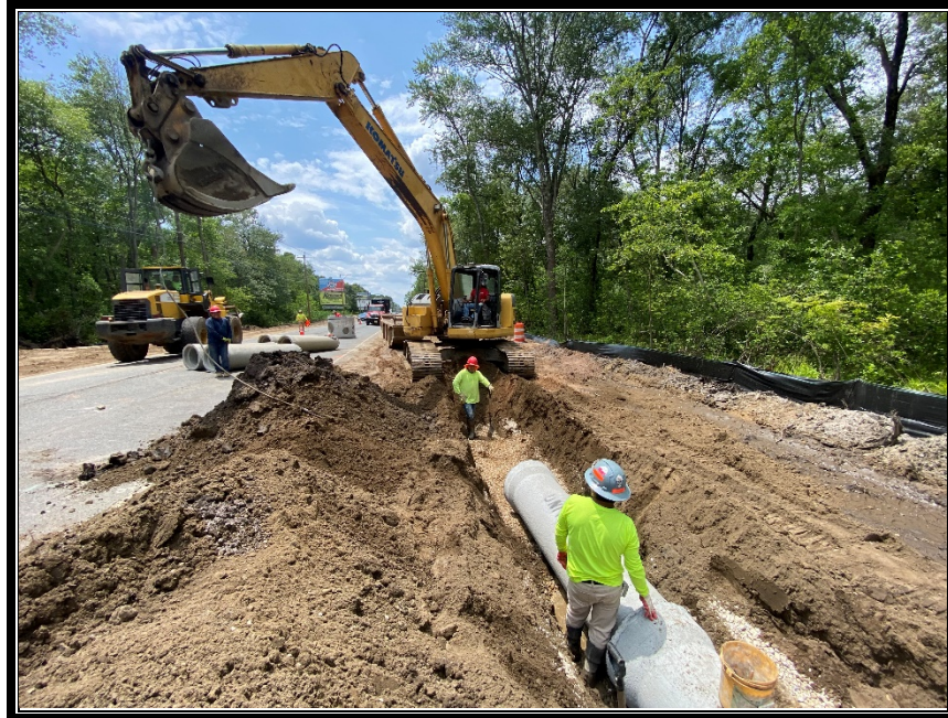
Figure 2: P&A Construction continues to install the reinforced concrete pipe.
