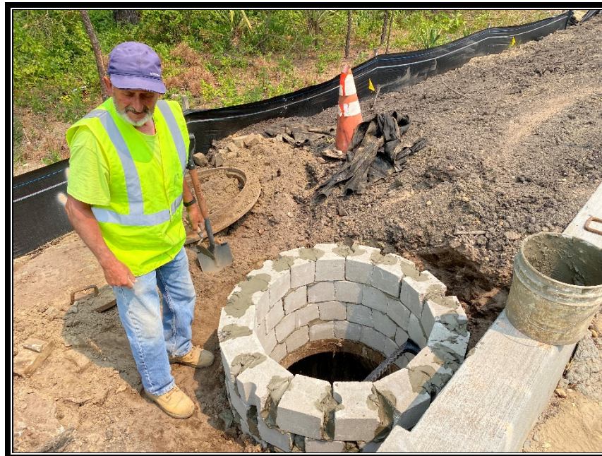
Figure 3: P&A Construction continues to raise existing and new structures to grade.
