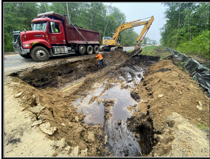
Figure 2: P&A Construction performing under-cutting.
