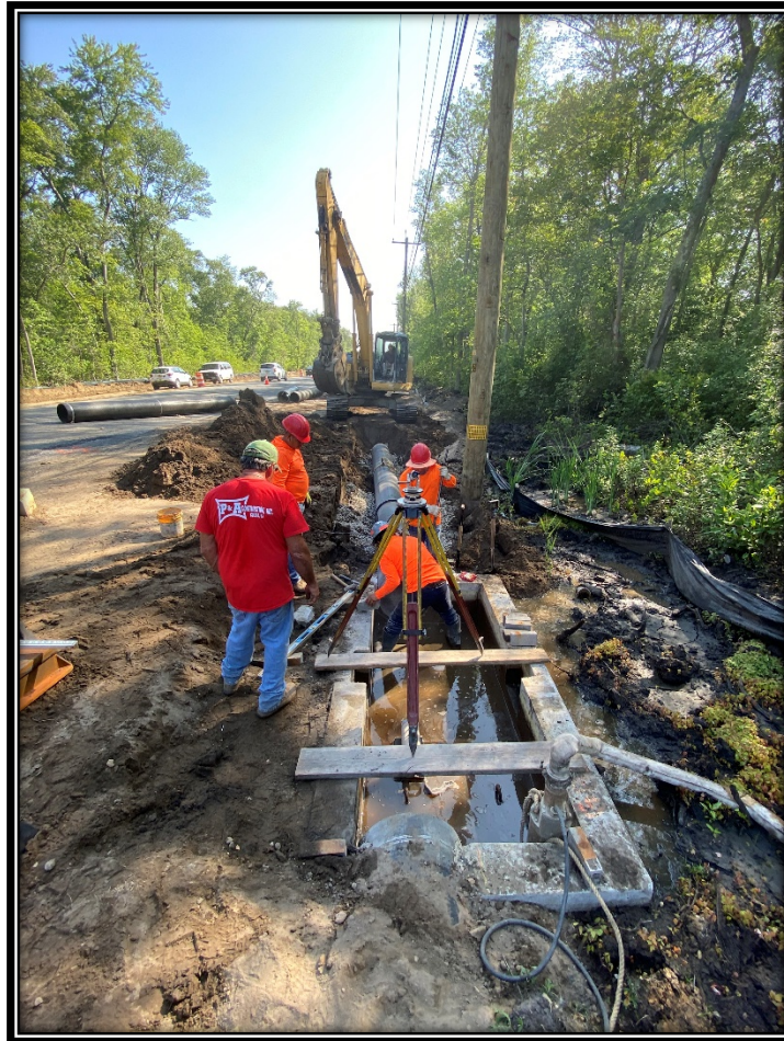
Figure: P&A Construction installing ductile iron pipe and inlet structures.
