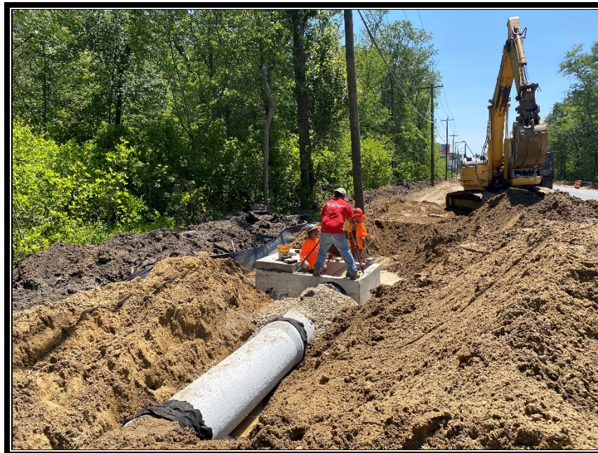
Figure 3: P&A Construction continues to install reinforced concrete pipe.
