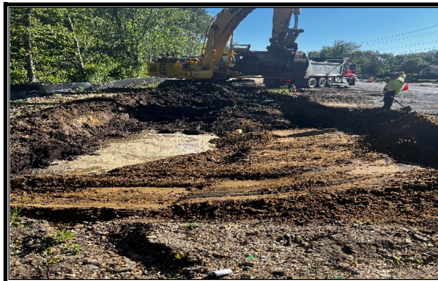
Figure 3: P&A Construction started the undercutting operation.
