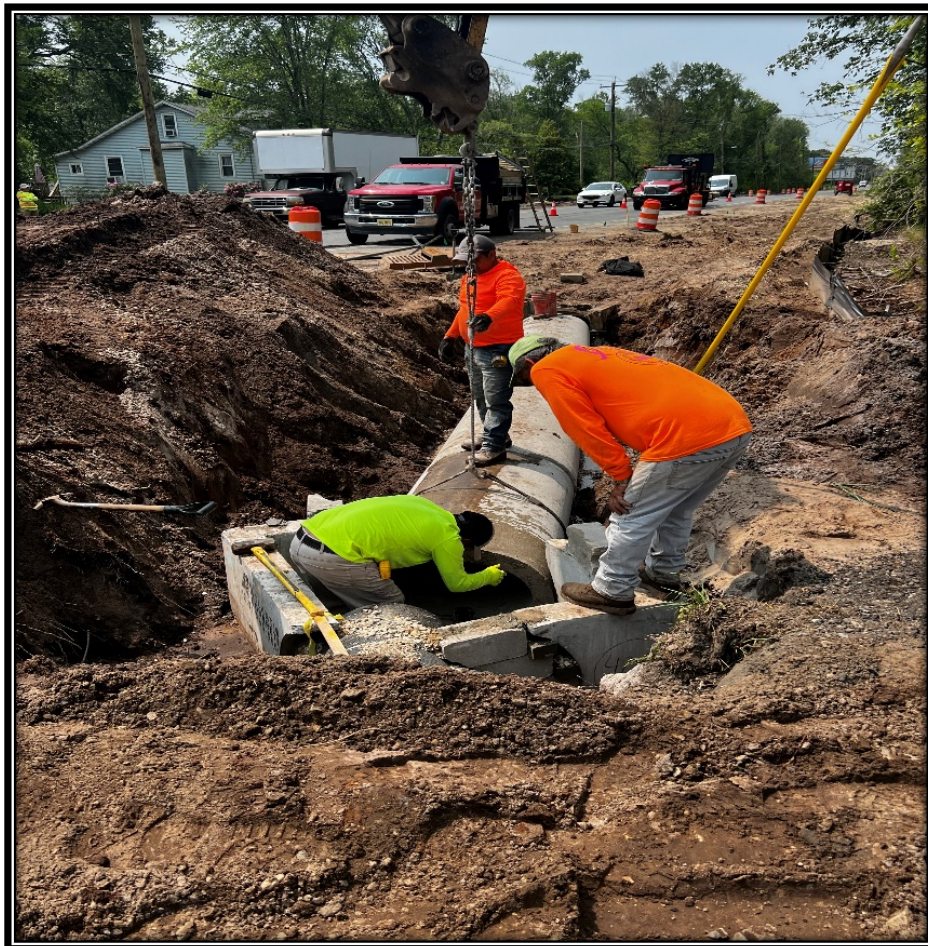
Figure: P&A Construction installing reinforced concrete pipe and inlet structures.
