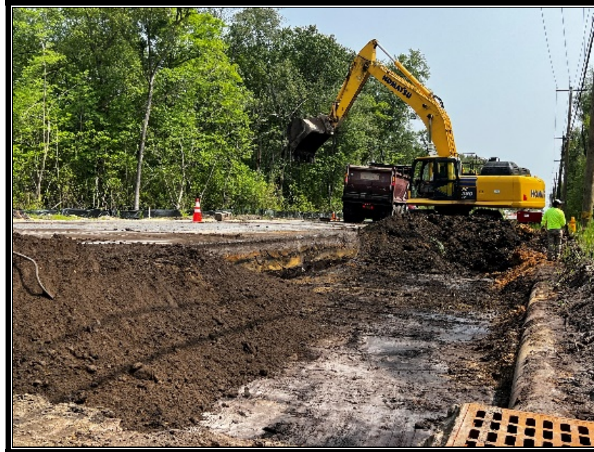
Figure 2: P&A Construction performing excavation unclassified.
