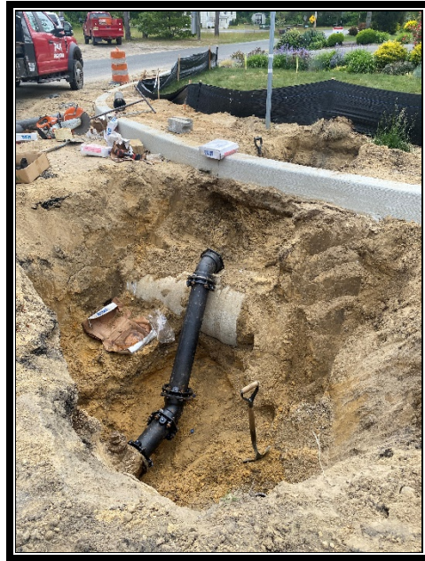
Figure 2: P&A Construction relocating hydrants.
