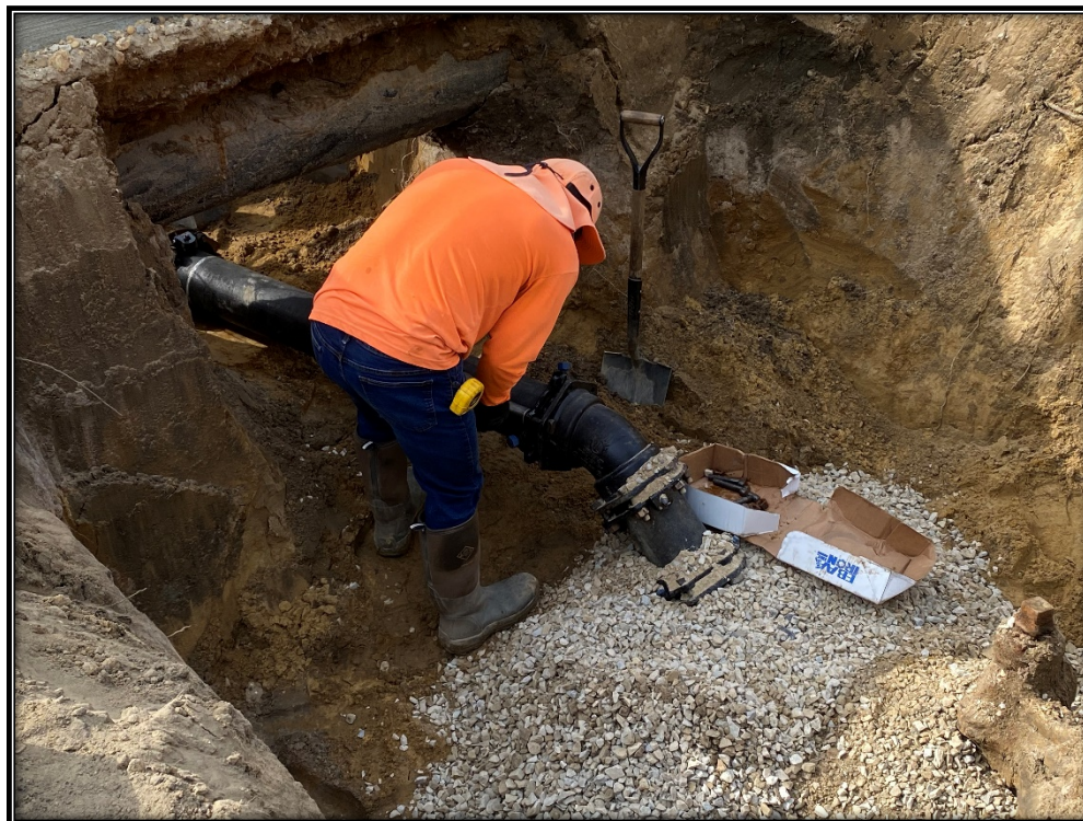
Figure: P&A Construction relocating hydrants.
