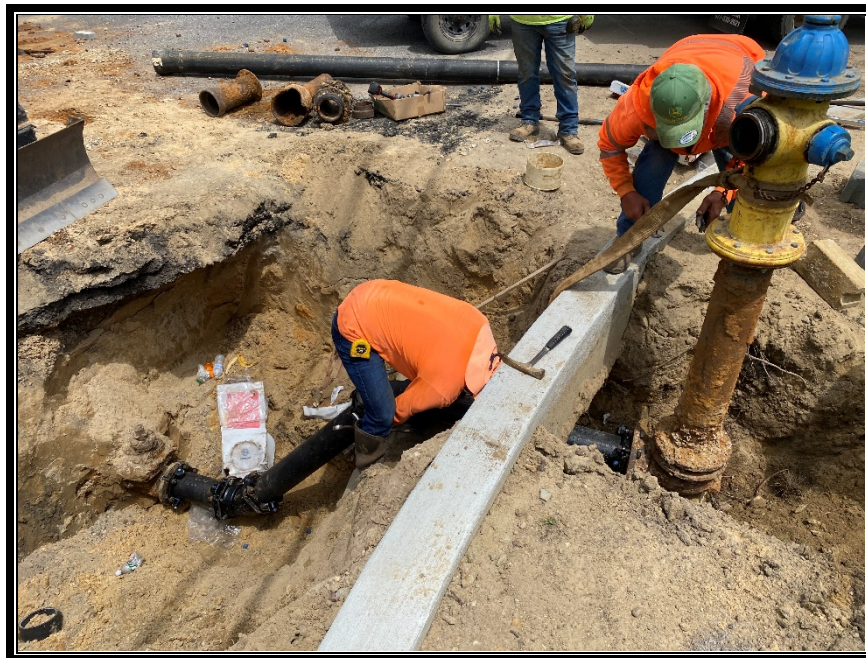
Figure 3: P&A Construction relocating hydrants.
