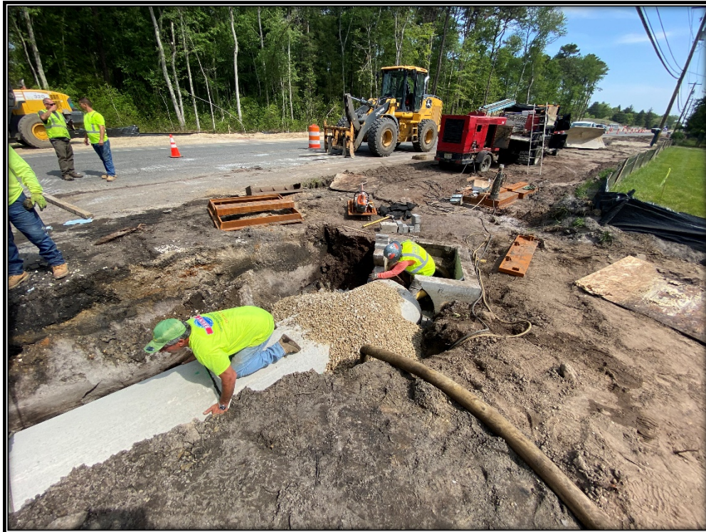
Figure: P&A Construction continues to install reinforced concrete pipe.
