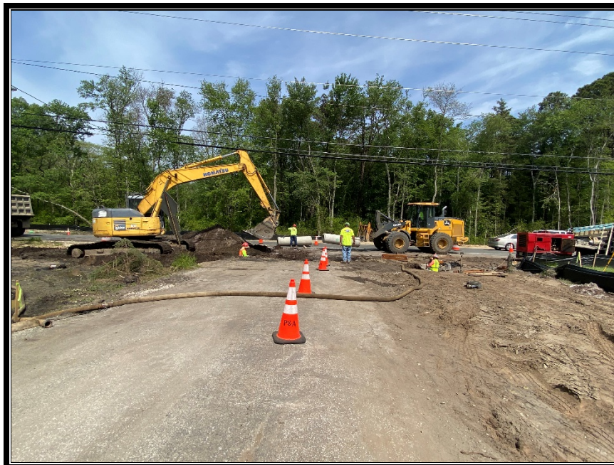
Figure 3: P&A Construction reinforced concrete pipe.
