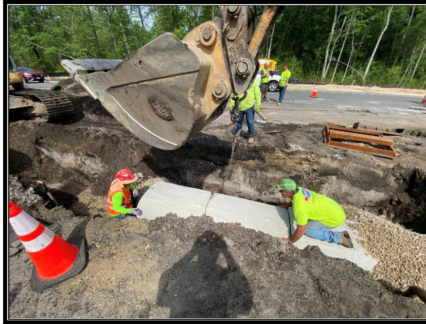
Figure 2: P&A Construction installing reinforced concrete pipe.
