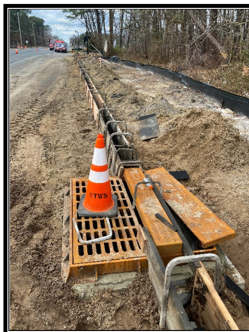
Figure 3: P&A Construction crew forming and pouring concrete curb.
