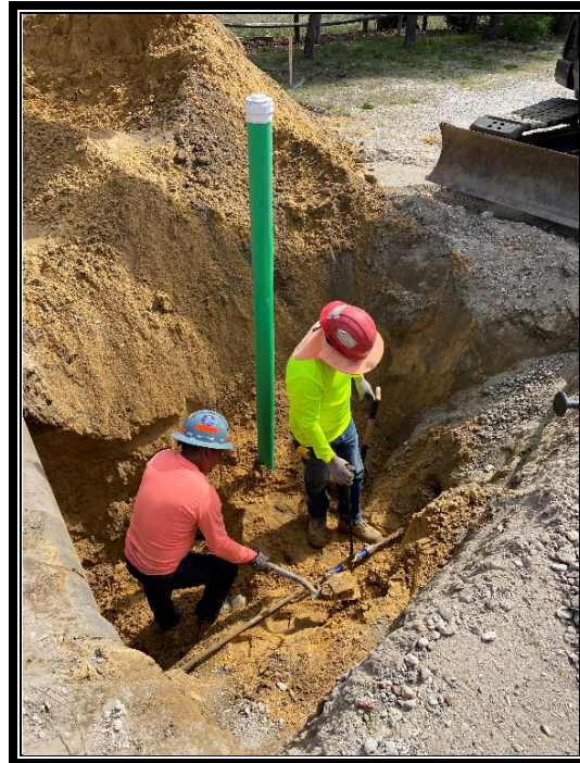
Figure 2: P&A Construction installing new sanitary sewer laterals and cleanouts.
