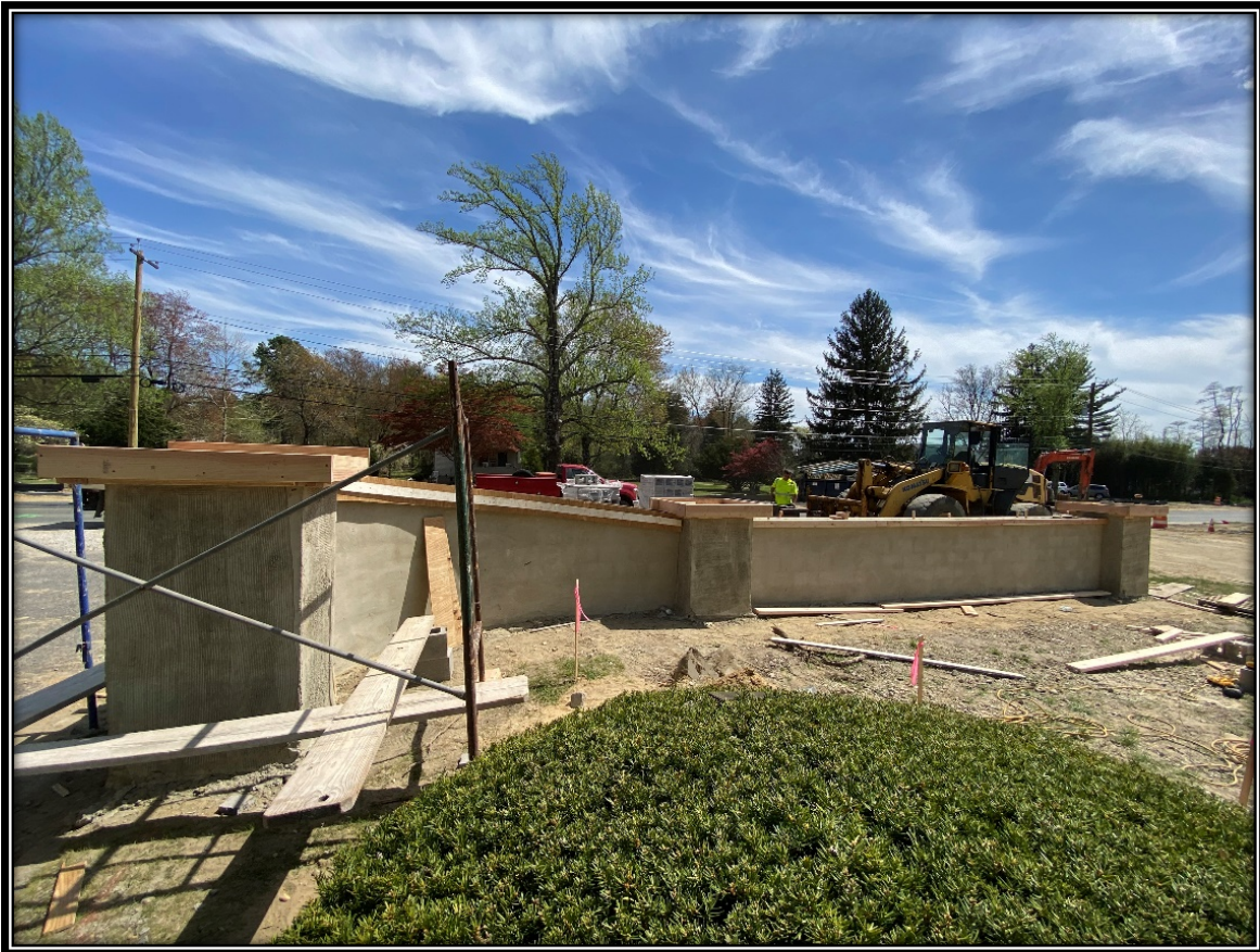
Figure: P&A Construction continues to reconstruction the decorative wall.
