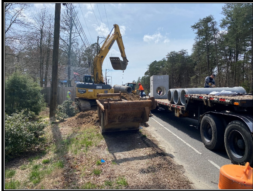
Figure 2: P&A Construction installing precast concrete structures.
