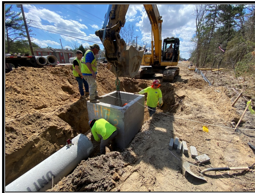
Figure 3: P&A Construction installing reinforced concrete pipe.
