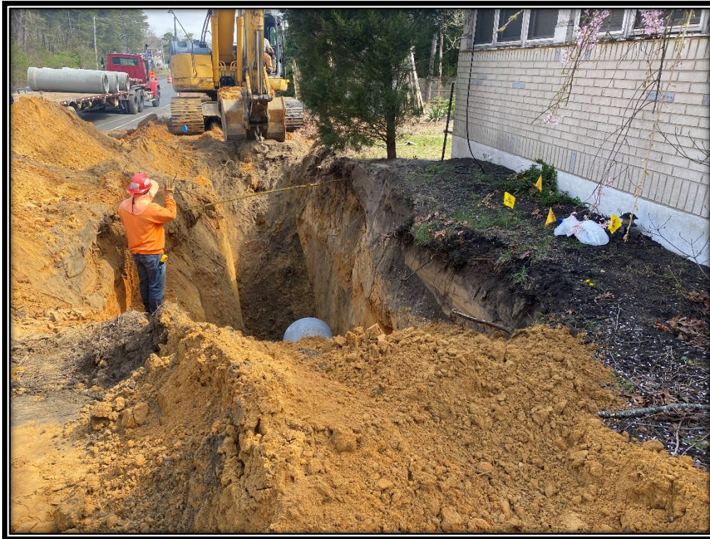
Figure: P&A Construction continues to install the reinforced concrete pipe.
