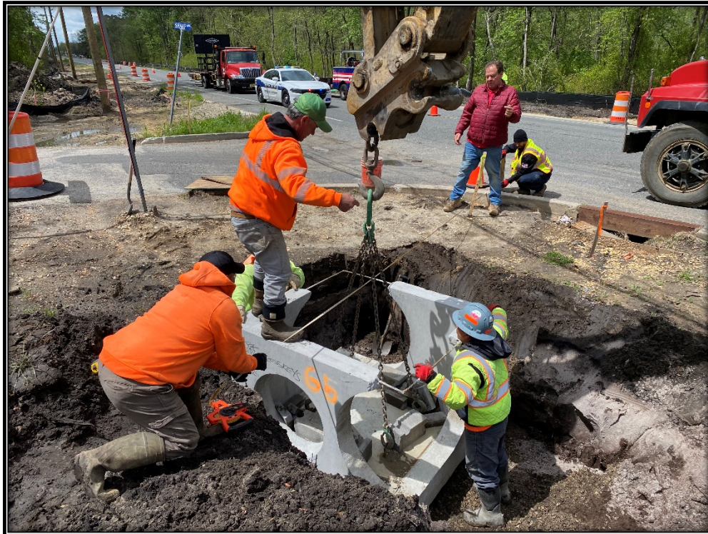
Figure: P&A Construction continues to install precast structures (inlets).
