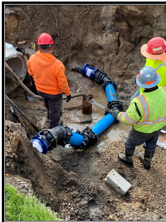
Figure 3: P&A Construction relocating 10" watermain.
