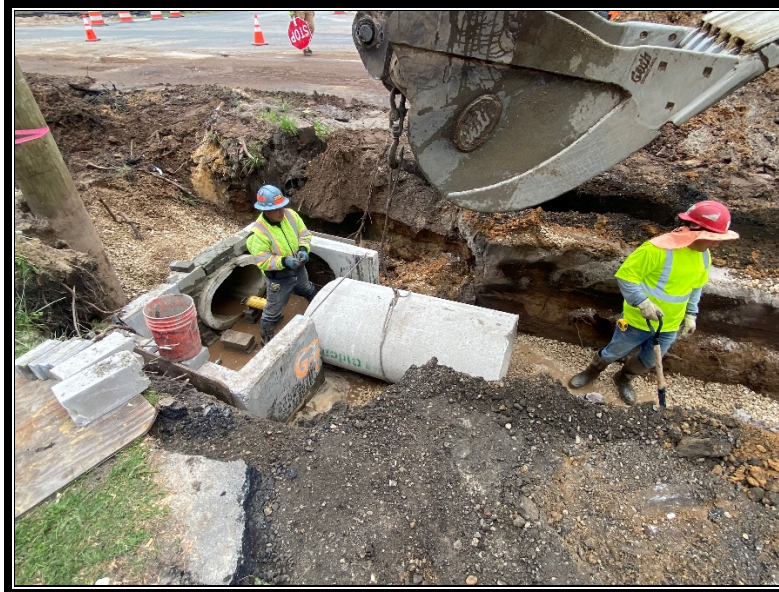
Figure 2: P&A Construction installing reinforced concrete pipe.
