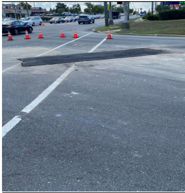
Figure 1: Asphalt patchwork
