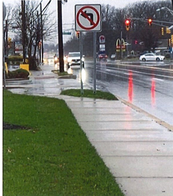
Figure 3: No Left Turn sign installed
