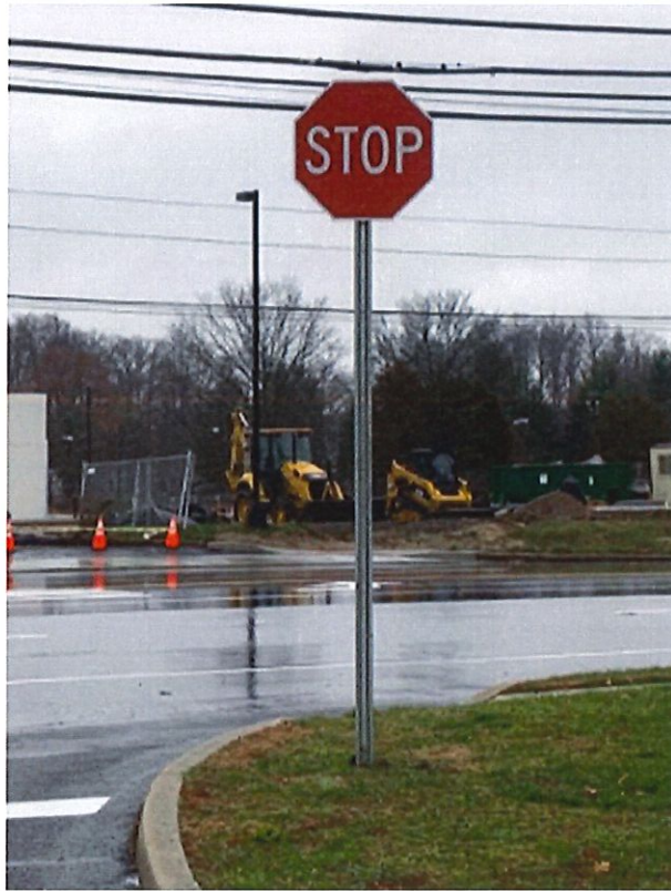
Figure 1: New Stop sign installed
