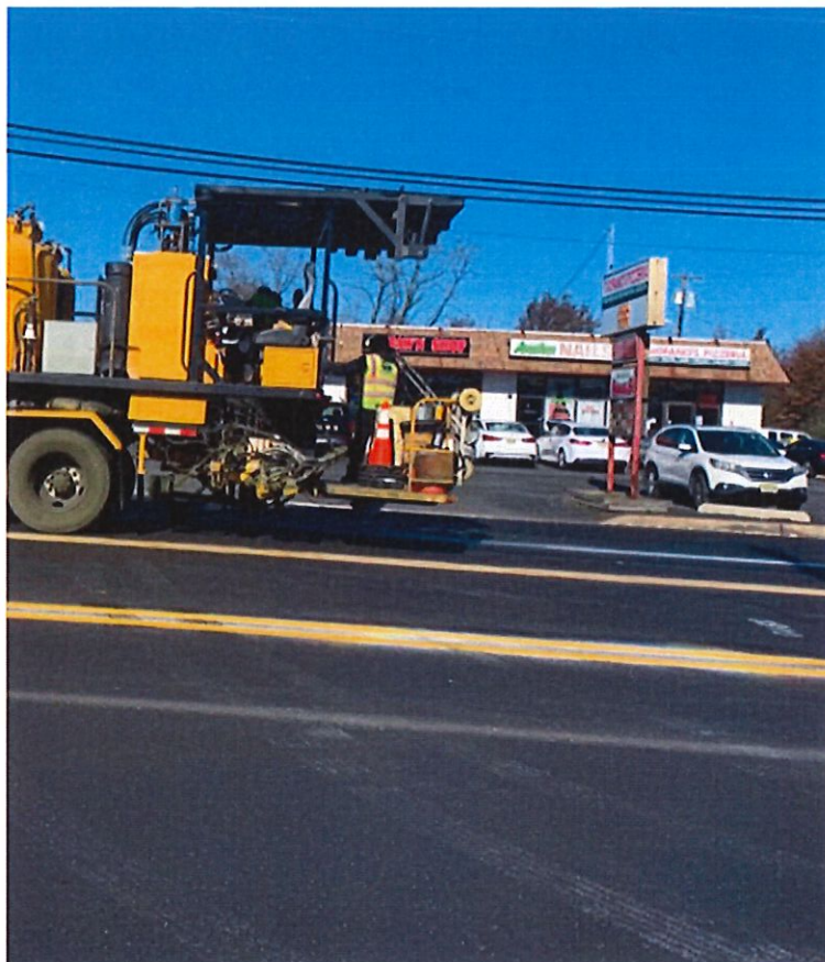
Figure 1: Epoxy striping in progress
