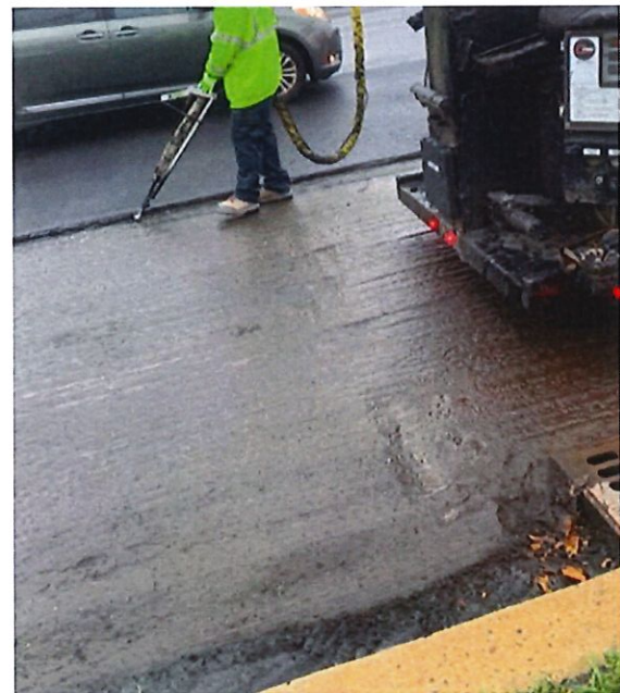
Figure 5: Polymerized Joint Adhesive applied
