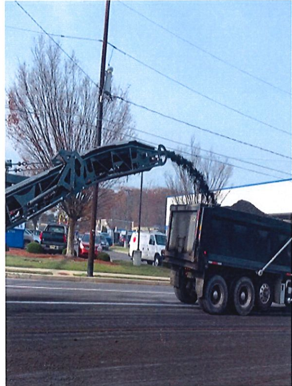
Figure 3: HMA Milling
