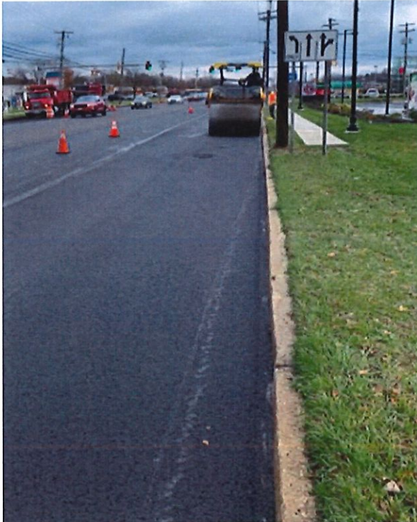
Figure 2: Compacting HMA
