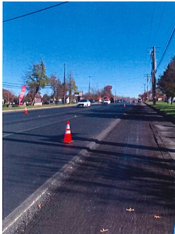
Figure 1: Milled roadway surface
