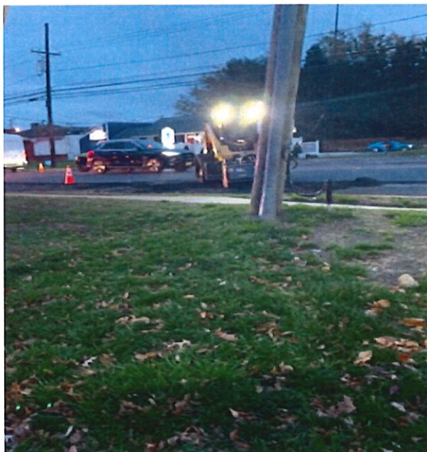
Figure 4: Box mill around manholes
