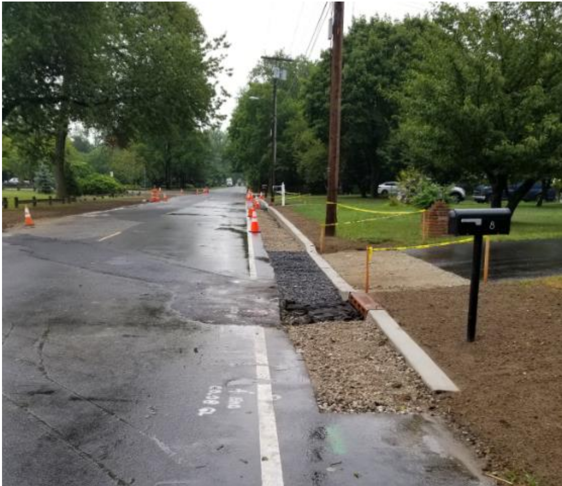
Figure: 1 – Concrete Curb construction at N. Park Drive.
