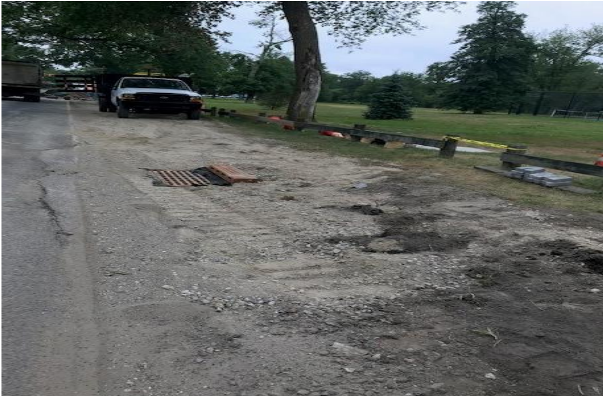
Figure: 2 – Inlet and Pipe replacements on N. Park drive near Lake
