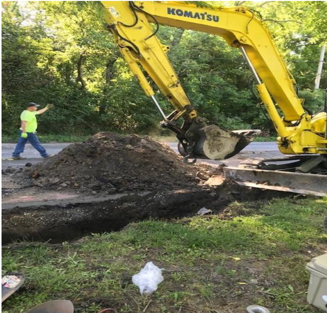
Figure: 1 – Utility pipe and Inlet replacement on N. Park Drive.
