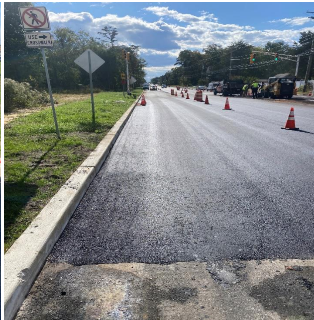
Figure 2: HMA Intermediate Course Placement
