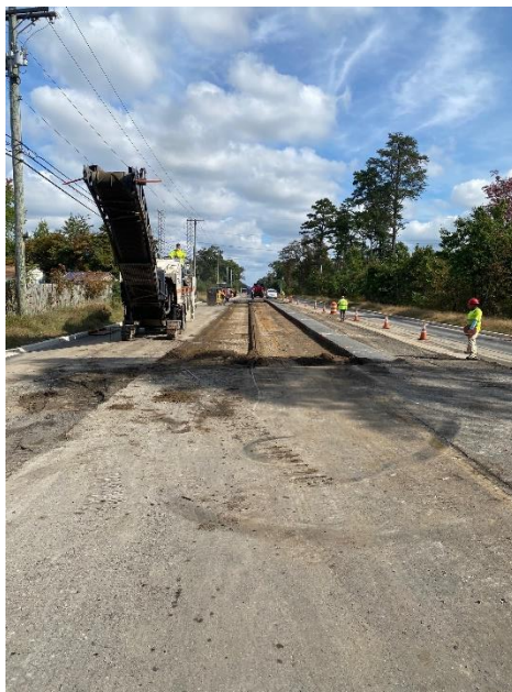
Figure 1: Milling/box out of BXKeys Road
