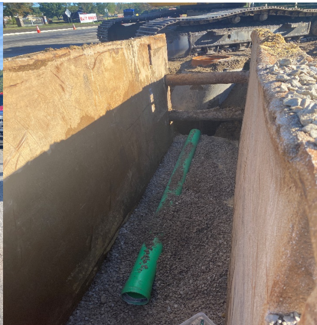
Figure 2: Sanitary Manhole/8" sanitary pipe installation
