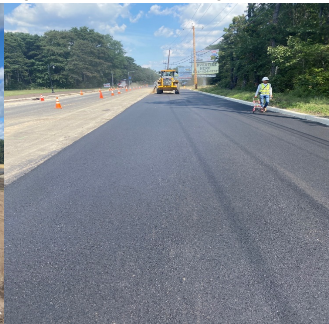
Figure 2: HMA Intermediate Paving (Station 60+00, RT)
