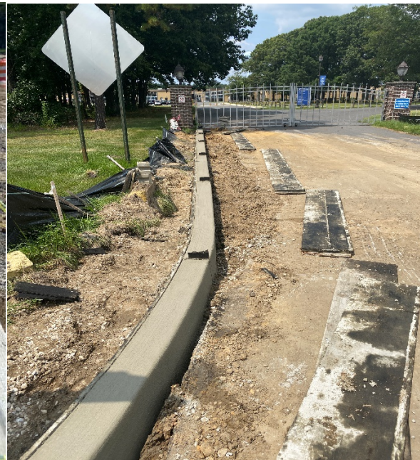
Figure 2: 9"X18" Concrete Vertical Curb Radius
