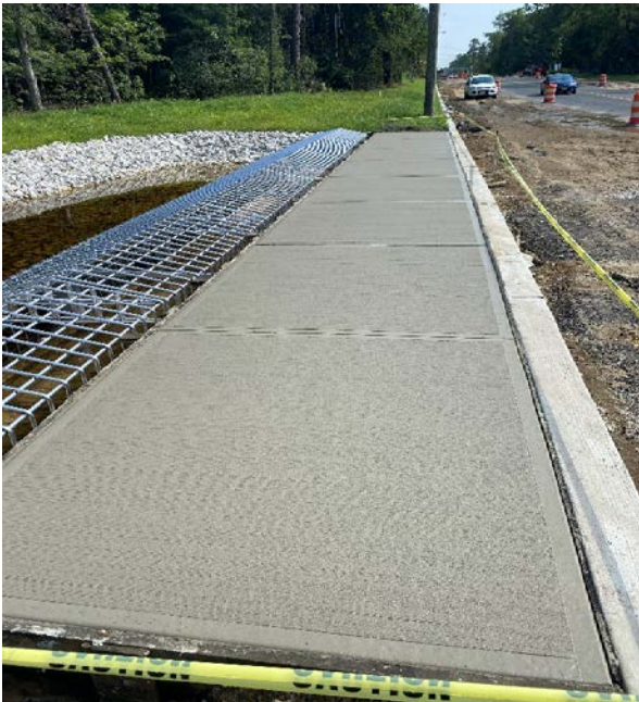
Figure 1: Reinforced Concrete Sidewalk, 8" Thick
