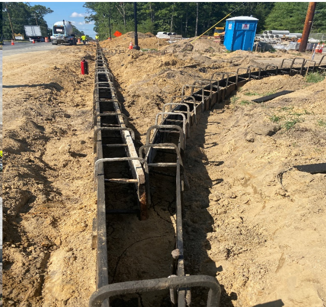
Figure 2: 9"X18" Concrete Vertical Curb Forms
