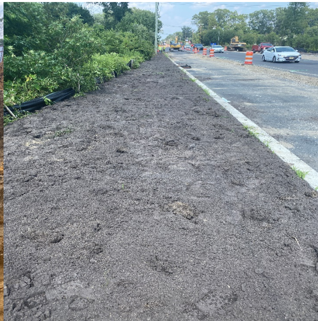
Figure 2: Topsoil/Seed Placement on Berlin Cross Keys Rd
