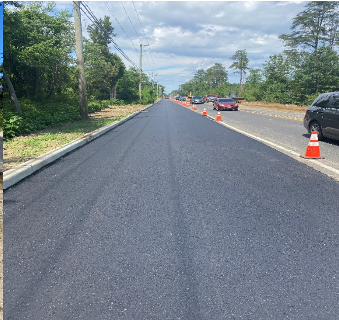
Figure 2: HMA 25M64 Base Paving
