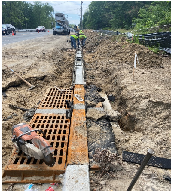
Figure 2: 9"X18" Concrete Vertical Curb Placement
