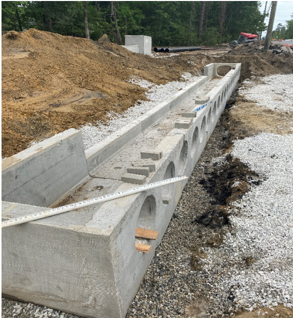
Figure 1: Dropbox installation for 20-18" Pipe Crossing Figure 2: HMA Paving over 20-18" DIP Crossing
