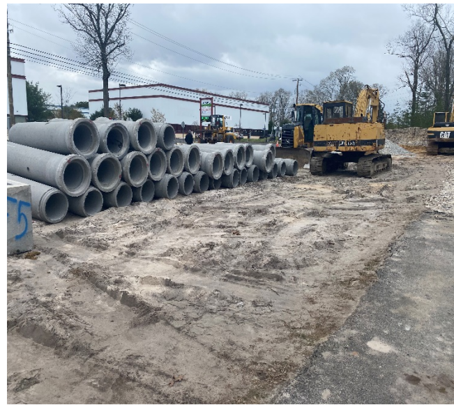
Figure 2: RCP/inlets delivered to job site
