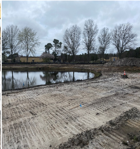
Figure 1: Headwall for pipe crossing near Old Bridge Rd Figure 2: Stripping of topsoil at CCTS pond
