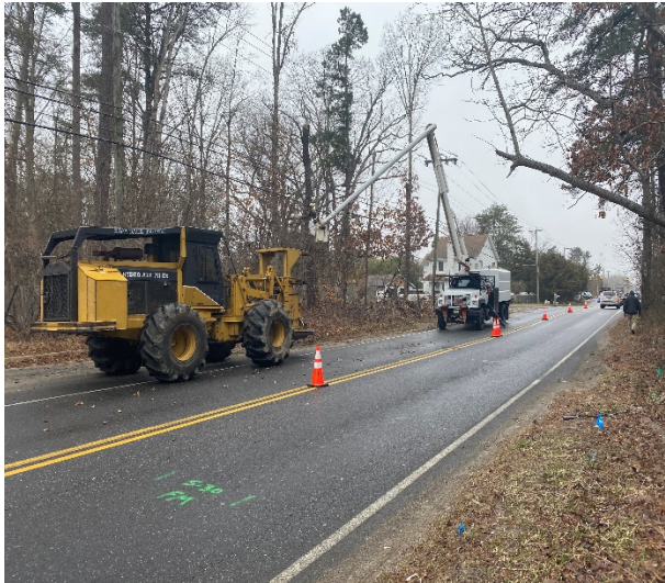
Figure 1: Stella Contracting clearing trees/brush
