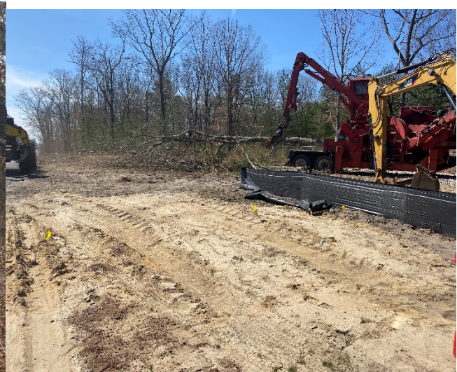
Figure 2: Stella Contracting sending trees through chipper
