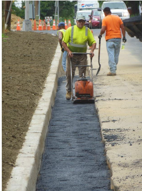
Figure 4 Bituminous material was placed in the front side of the newly installed curb
