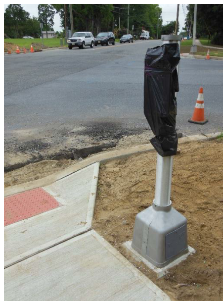
Figure 5 Contractor graded and dressed up the area where new Push button poles were installed
