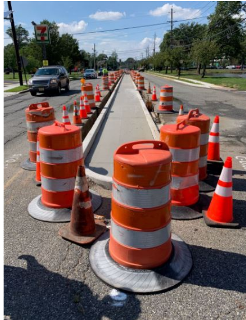
Figure 1: Concrete center island construction
