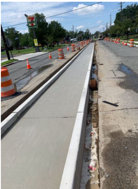
Figure 2: Concrete center island paver base
