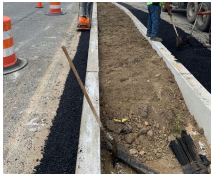
Figure 3: Center island roadway restoration
