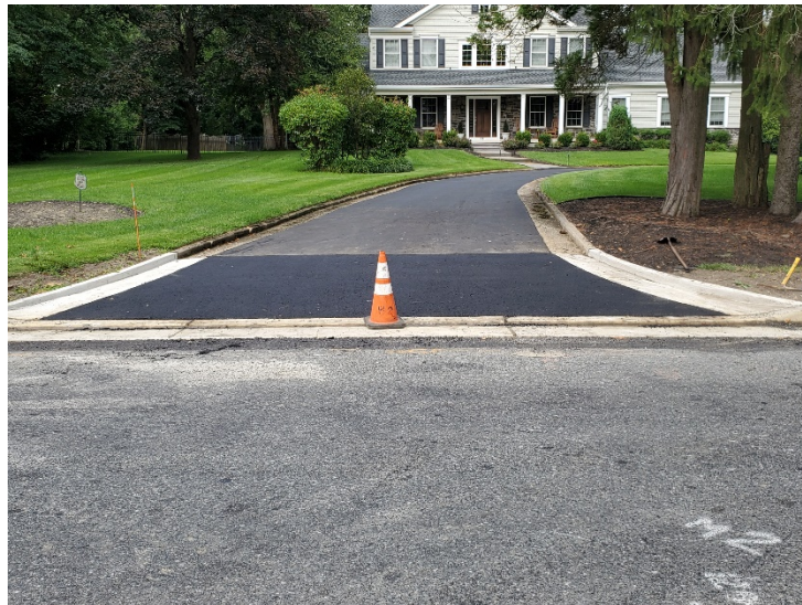
Figure 3 Hot mix asphalt driveway completed at Sta. 129+00 and 130+00 (both left offsets)
