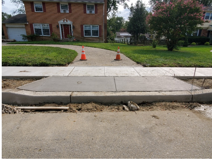
Figure 4 Concrete driveway with welded steel wires constructed along EB Kresson Road
