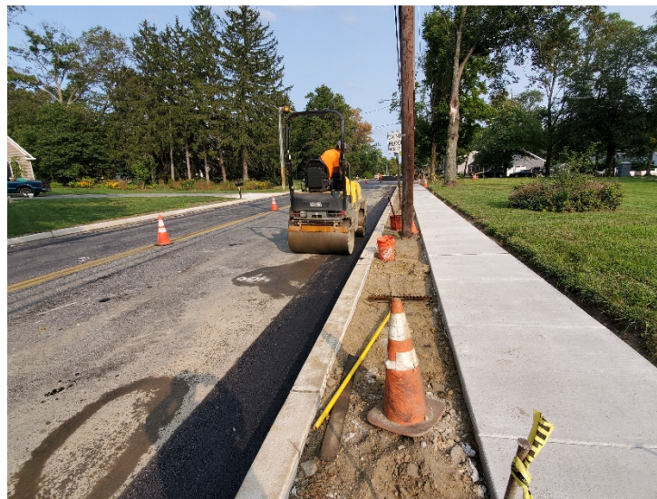
Figure 5 Curb restoration using hot mix asphalt done along EB Kresson Road
