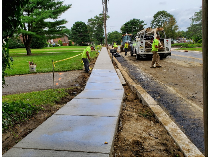
Figure 2 Concrete sidewalk constructed along EB Kresson Road
