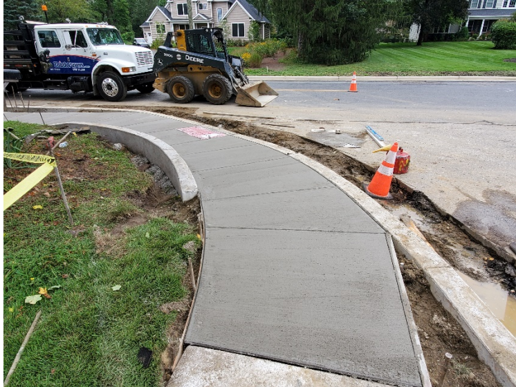
Figure 2 Curb ramp constructed at Sta. 128+20 (right offset)
