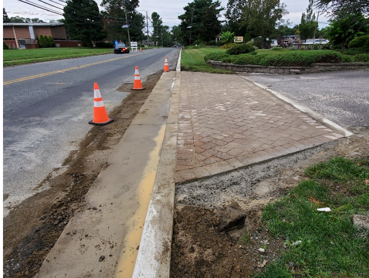
Figure 6 Driveway which included adding concrete base and resetting pavers at Sta. 121+10 (left offset)
