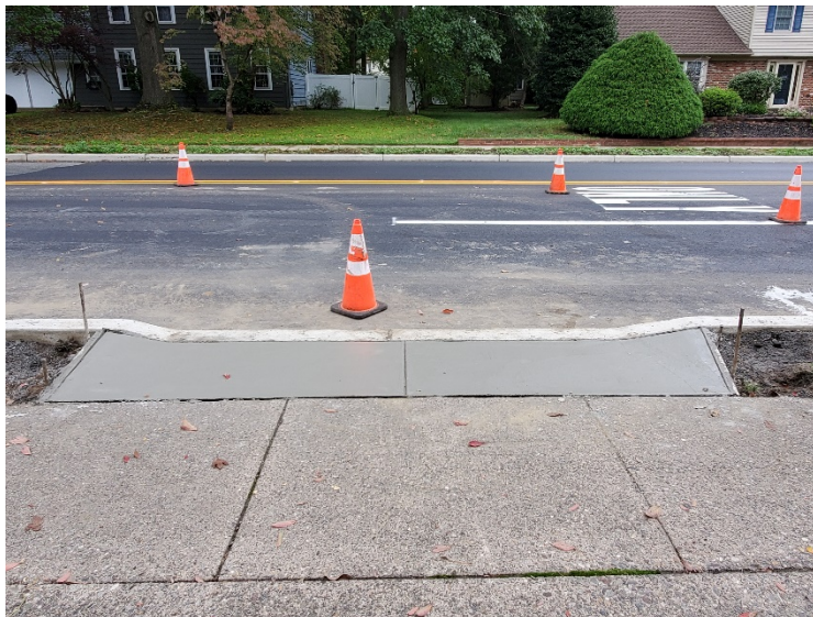
Figure 7 Concrete driveways with welded steel wires constructed along EB Kresson Road
