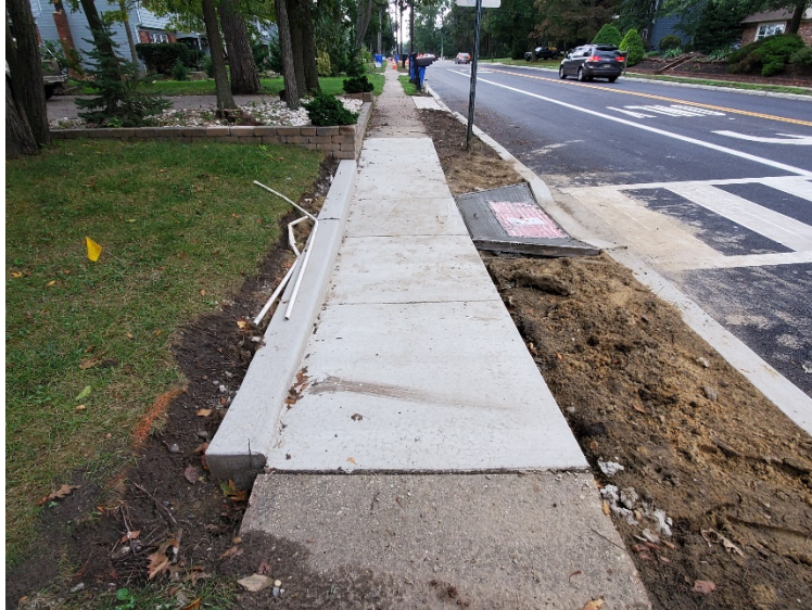
Figure 4 Curb ramp constructed at Sta. 132+83 (right offset)
