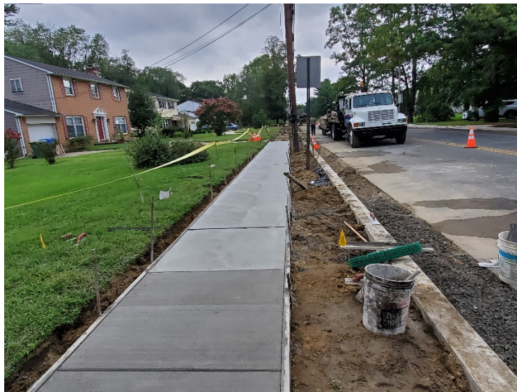
Figure 5 Existing concrete sidewalk removed and replaced along EB Kresson Road
