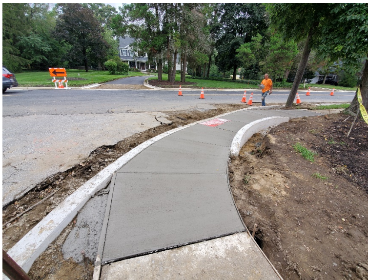
Figure 3 Curb ramp constructed at Sta. 129+09 (right offset)
