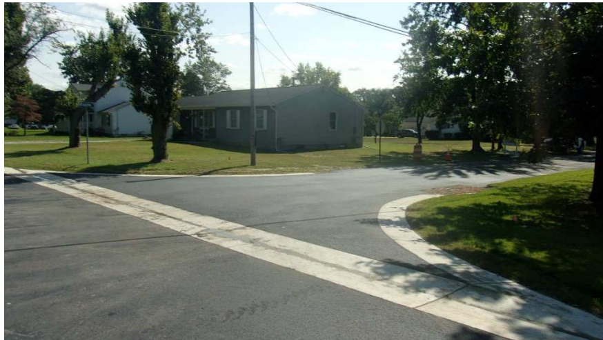
Figure 7 Placement of HMA surface course Maple Avenue.
