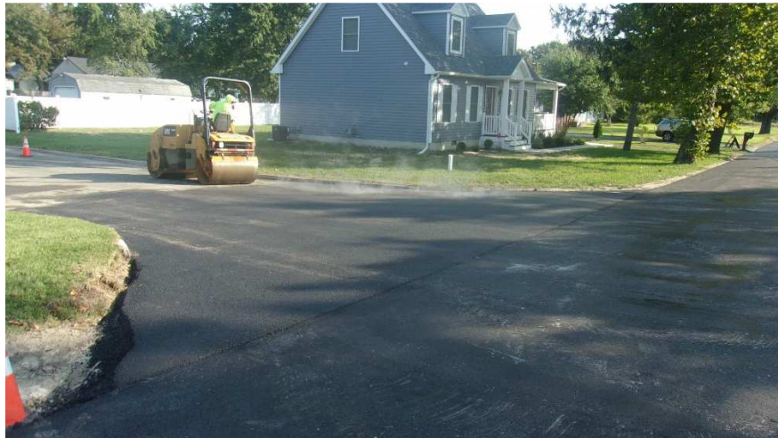
Figure 5 Placement of HMA surface course North Second Street.
