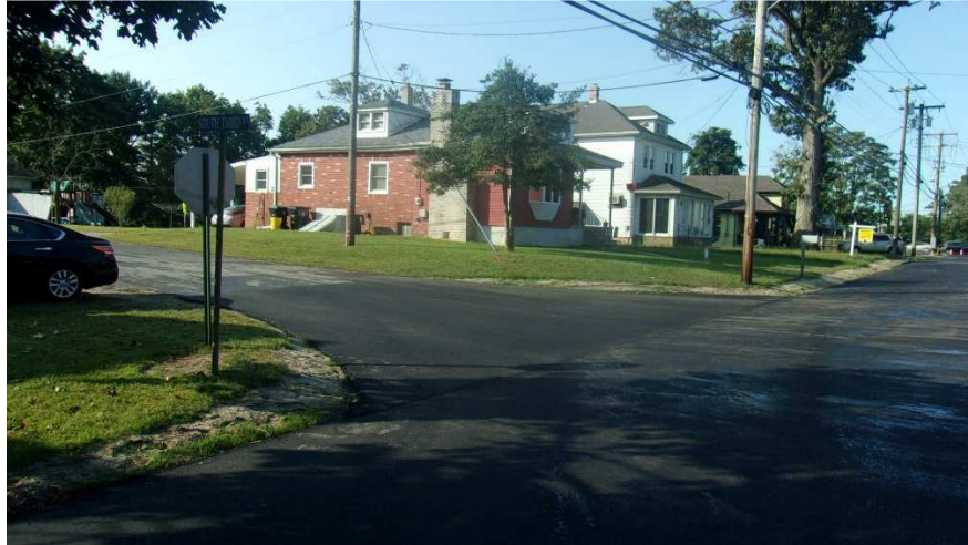
Figure 4 Placement of HMA surface course South Third Street.
