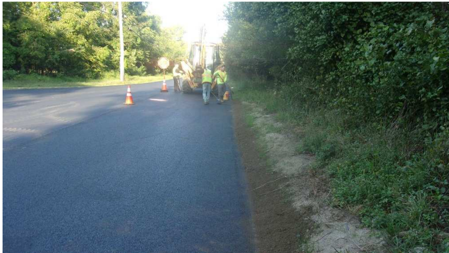
Figure 13 Reworked turf repair strip along Chew Road.
