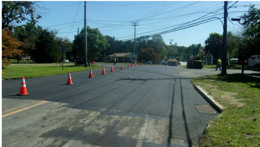
Figure 11 Placement of HMA surface course Old White Horse Pike intersection with Pennington Ave and Chew Road.
