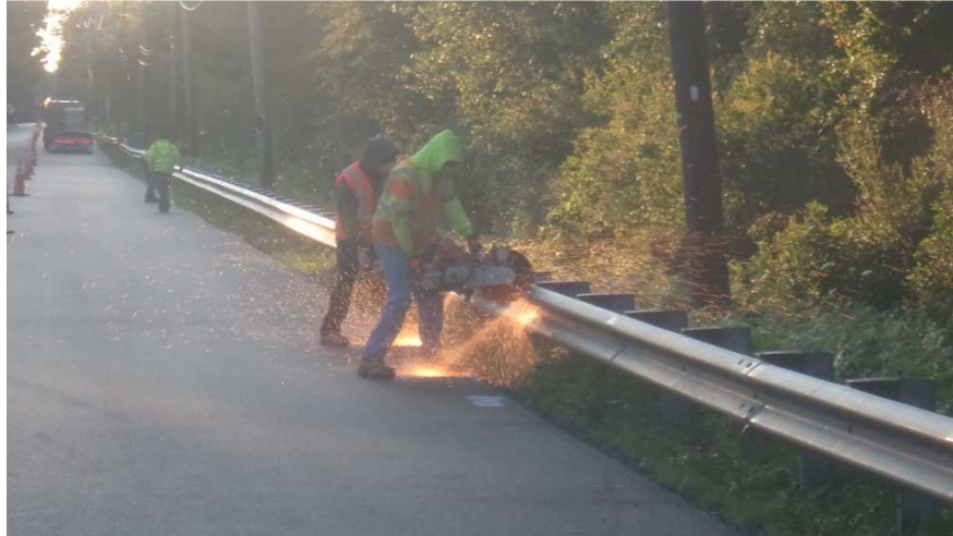
Figure 10 Removal of existing guide rail along Chew road.
