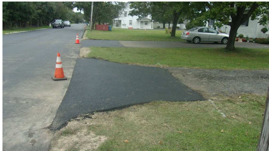
Figure 15 Typical HMA driveway installation along Chew Road.
