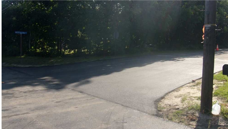
Figure 6 Placement of HMA surface course South Third Street.
