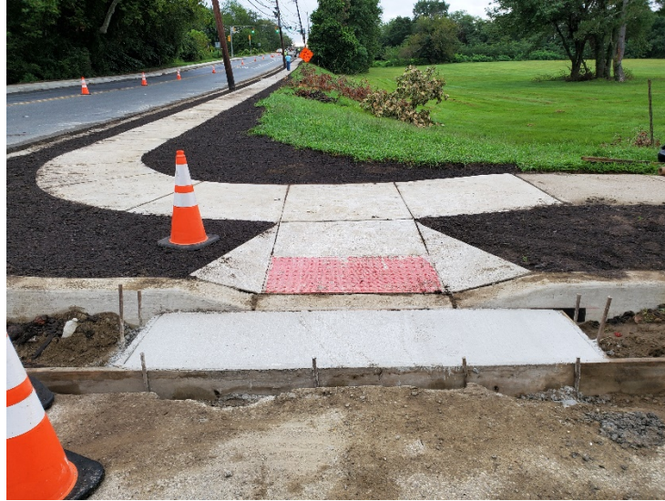
Figure 2 Curb ramp and concrete gutter constructed at Sta. 140+27 (right offset)
