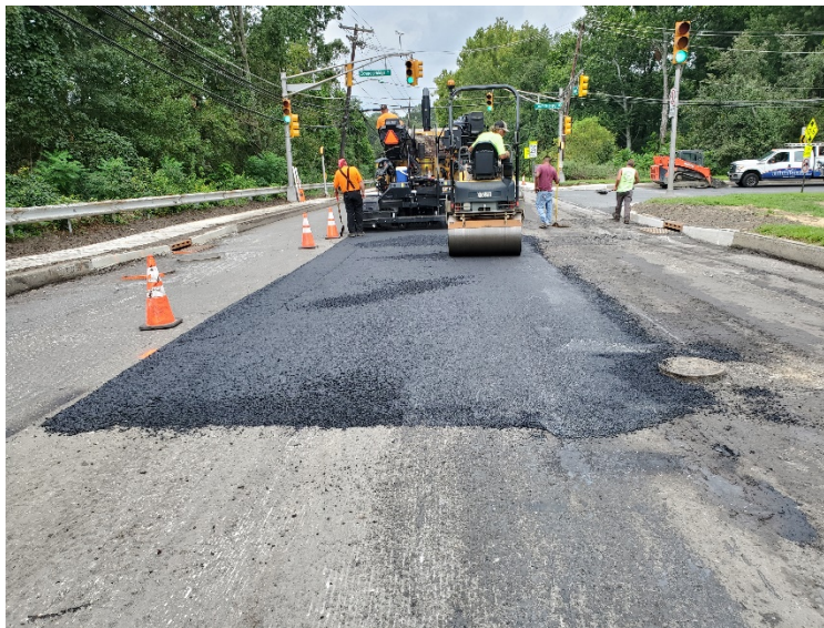
Figure 7 Asphalt level course 1/2" thick applied from Sta. 141+50 to 145+30 to cover the ballast until HMA paving
