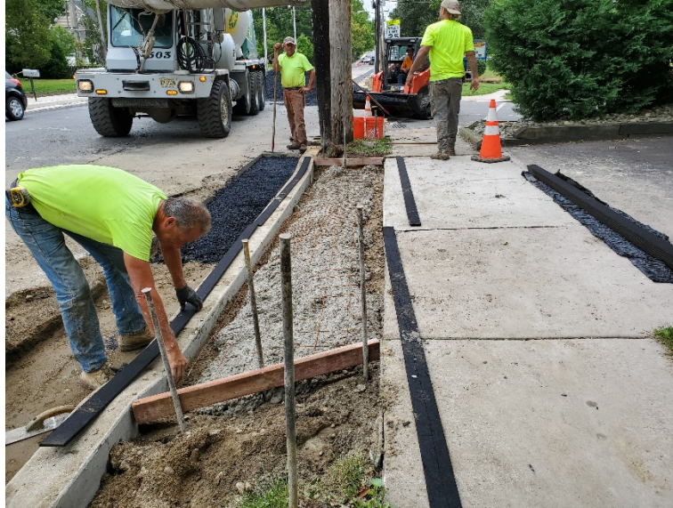
Figure 4 Concrete driveway constructed at Sta. 131+70 and 132+50 (both right offset)
