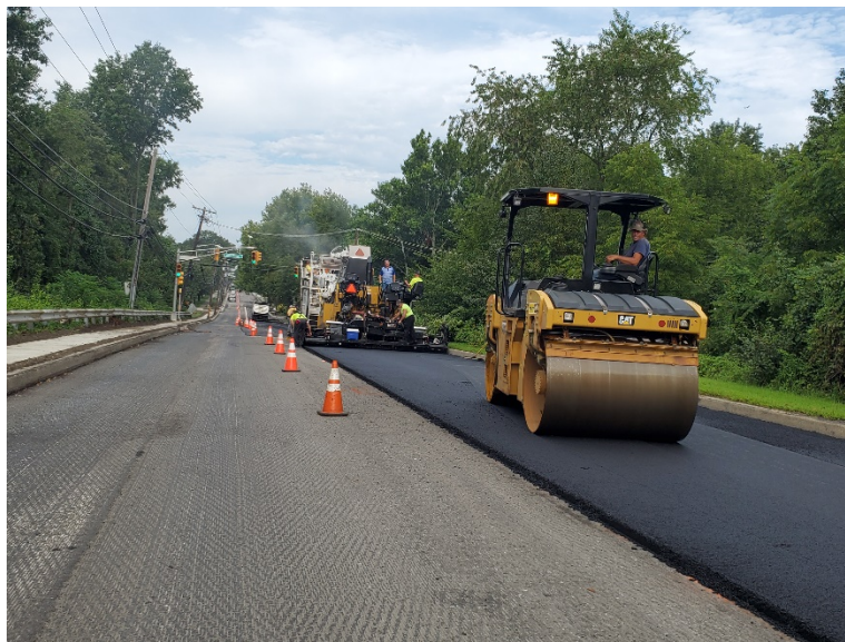
Figure 9 HMA paving on WB lane of Kresson Road
