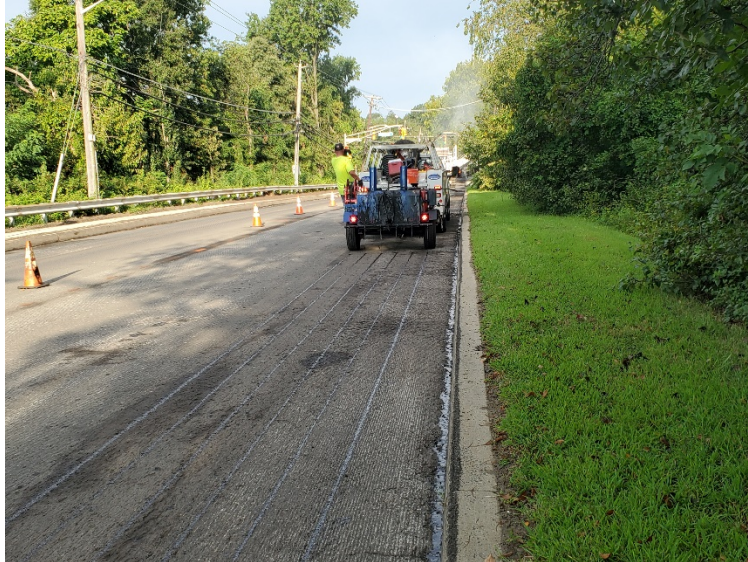
Figure 8 Tack coat applied prior to HMA paving
