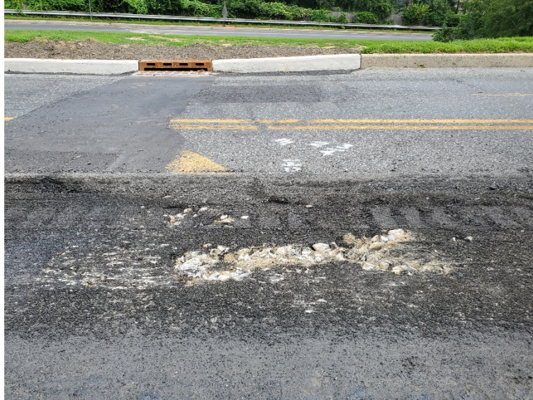
Figure 6 Ballast uncovered during HMA milling from Sta. 143+00 to 145+30 at the crown of the road
