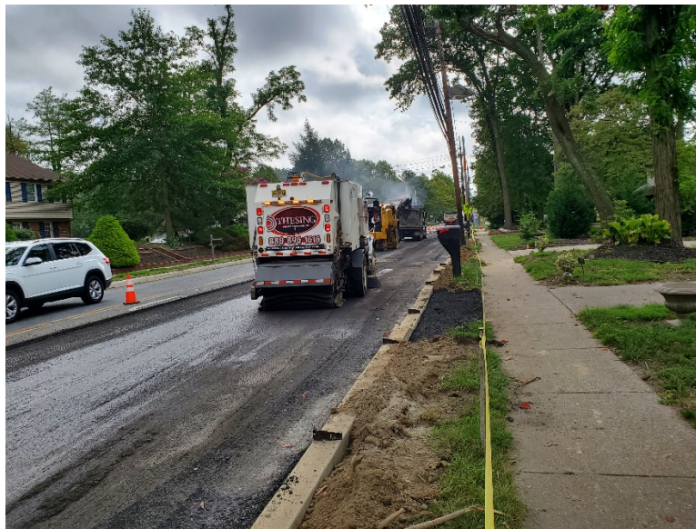
Figure 5 HMA milling and sweeping performed in both lanes of Kresson Road from Sta. 131+05 to 147+78
