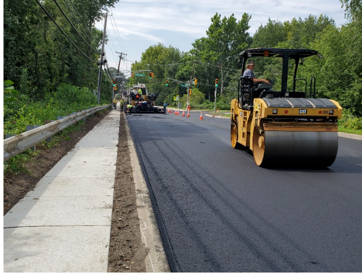
Figure 9 HMA paving on EB lane of Kresson Road
