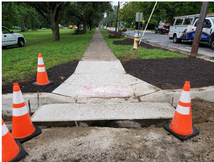
Figure 3 Curb ramp and concrete gutter constructed at Sta. 140+06 (right offset)
