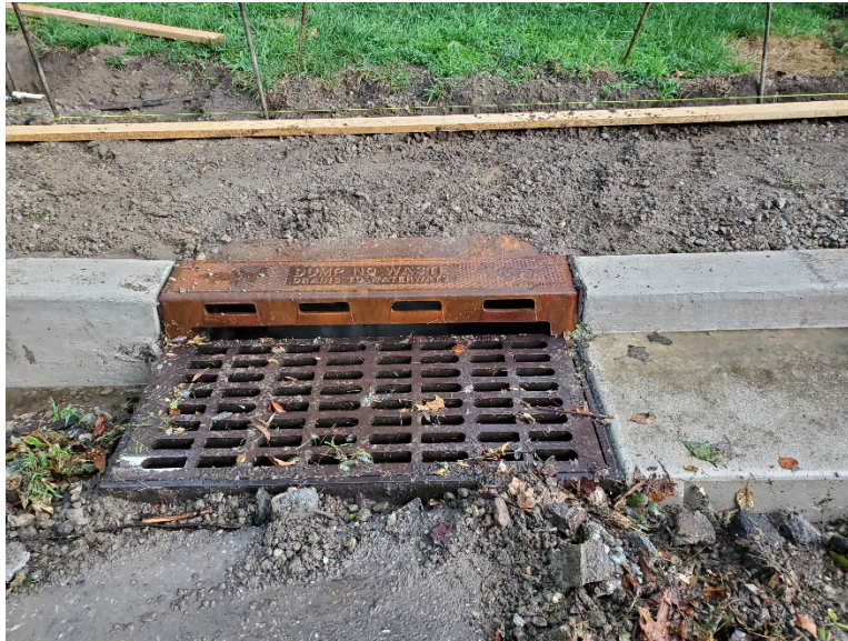
Figure 4 Curb piece, eco type 'N' installed at Sta. 133+55 (left offset)
