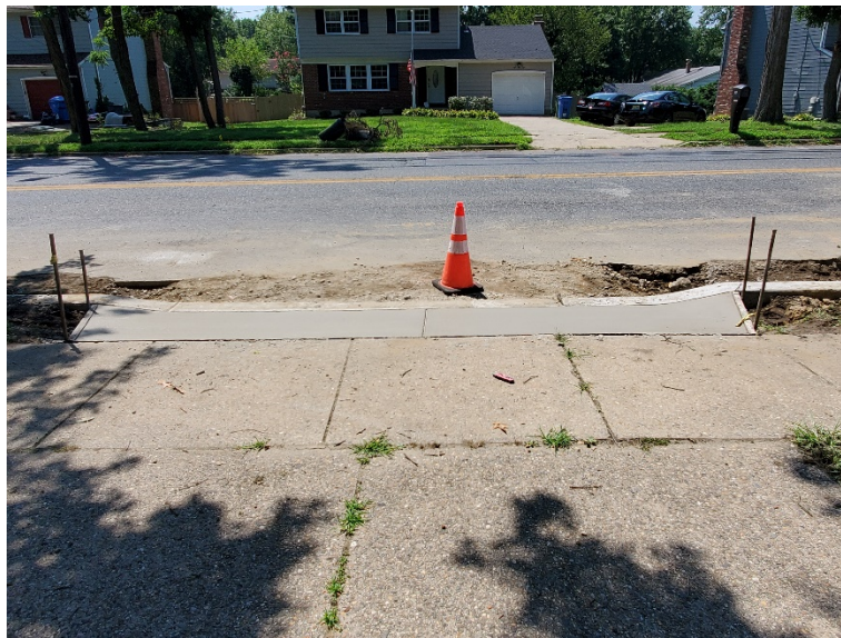
Figure 5 Concrete driveway, 6" thick with welded steel wire constructed at Sta. 130+65 (left offset)
