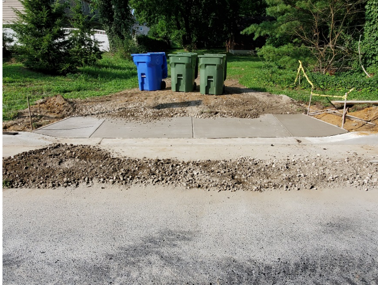
Figure 6 Concrete driveway, 6" thick with welded steel wire constructed at Sta. 137+10 (left offset)
