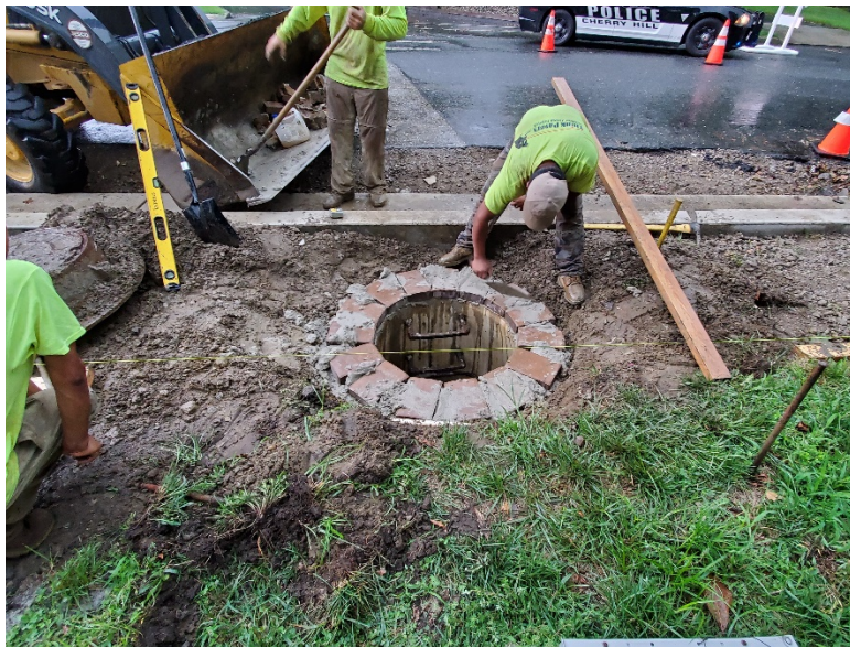
Figure 7 New bricks laid to lower existing manhole casting in the sidewalk of Sta. 133+70 (left offset)
