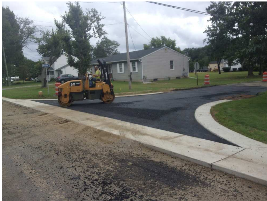
Figure 5 Maple Ave. base paved behind gutter.
