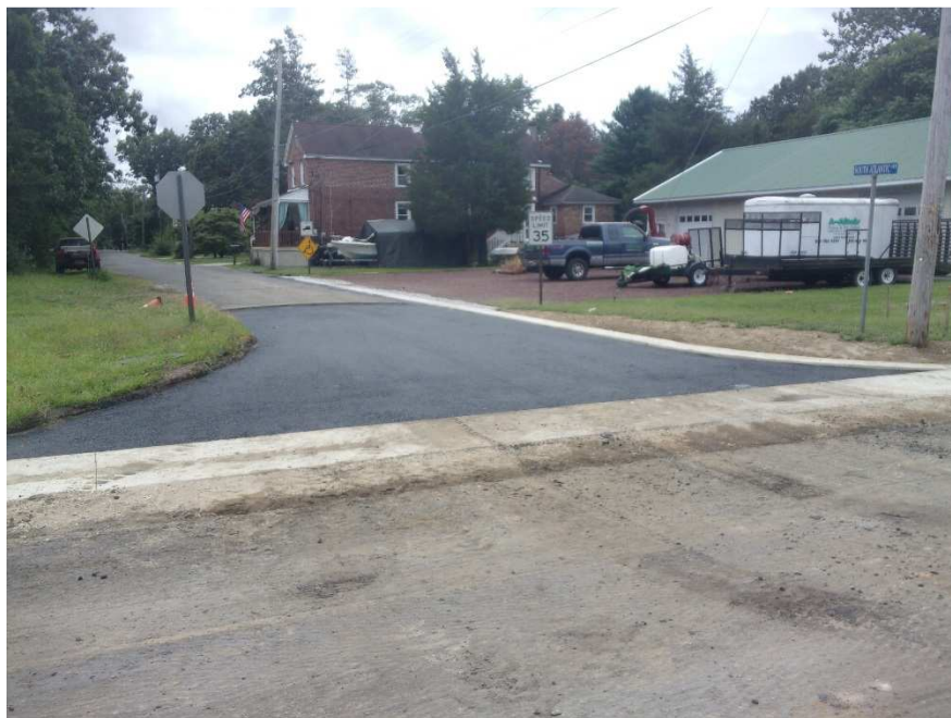
Figure 7 South Atlantic Street base paved behind gutter.
