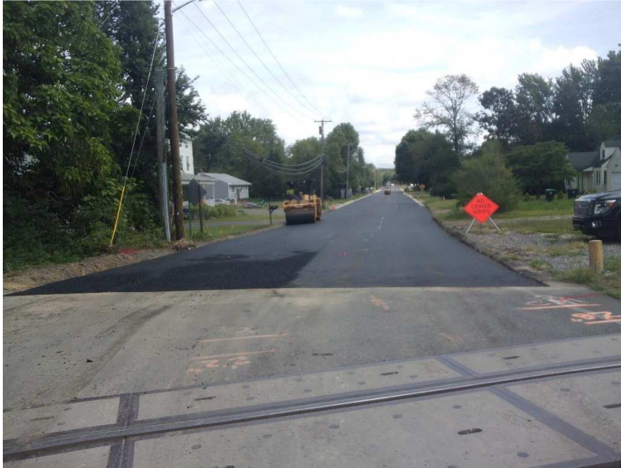
Figure 8 Base paving Pennington Ave. East of Railroad tracks
