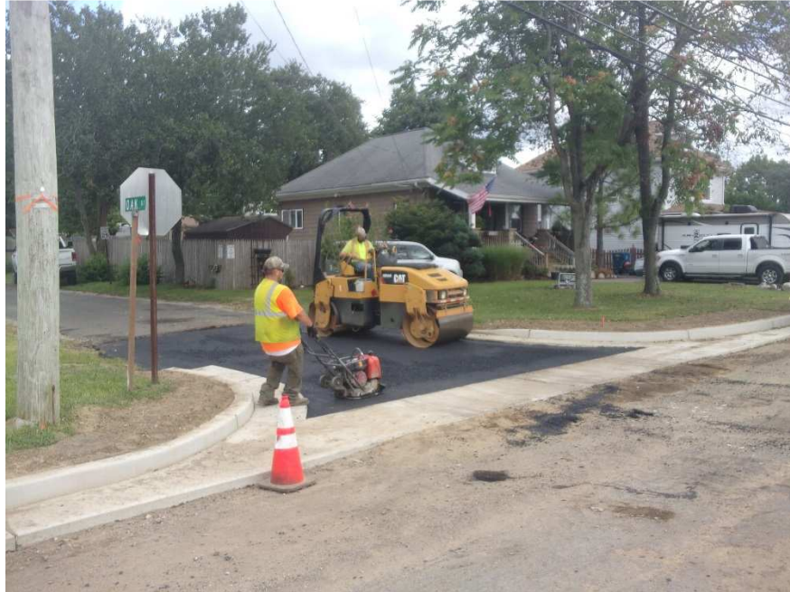
Figure 4 Oak Street base paved behind gutter.
