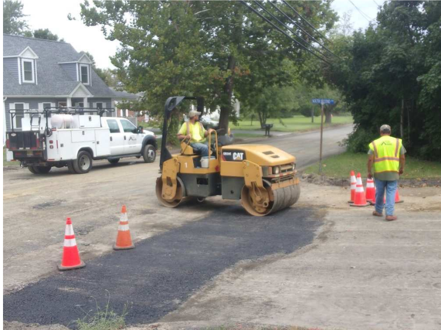
Figure 6 South Second Street base repair.
