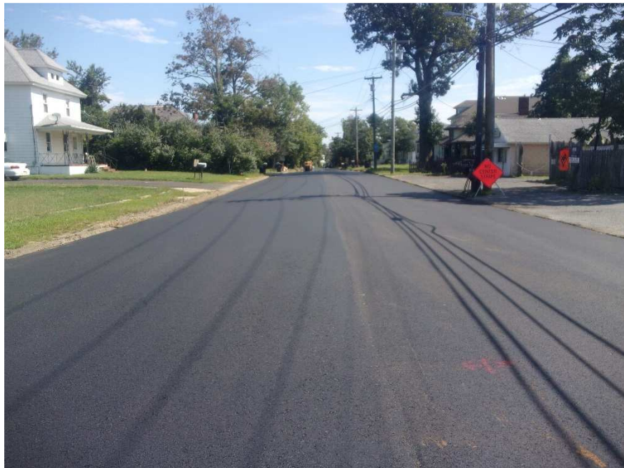
Figure 9 Base paving Pennington Ave. West of Railroad tracks
