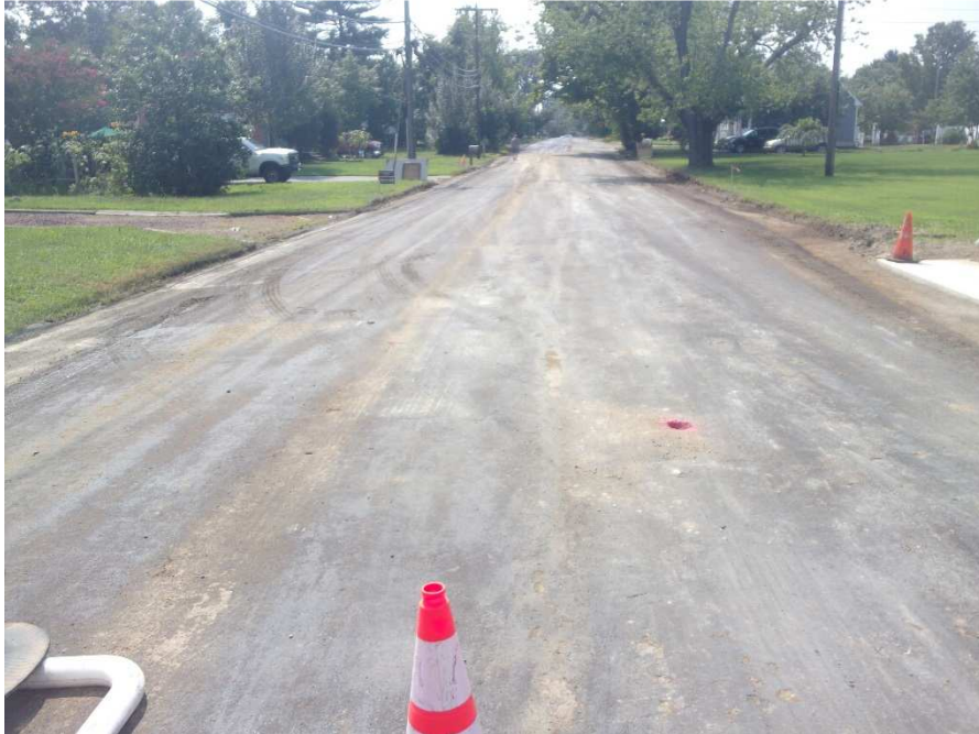
Figure 2 Full depth reclamation Pennington Ave. railroad looking towards Second Street
