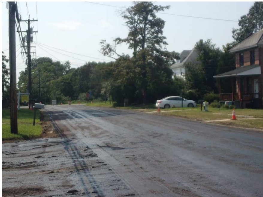
Figure 3 Full depth reclamation Pennington Ave. South Third Street looking towards Rout 30 White Horse Pike.
