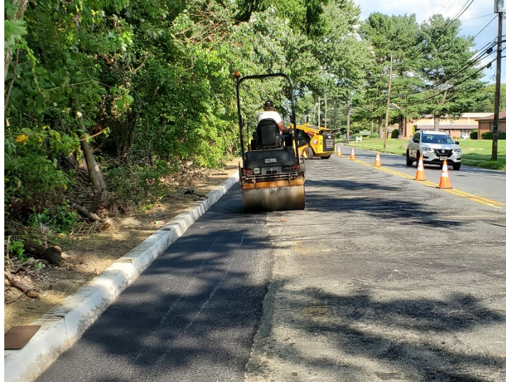
Figure 10 8" HMA used with temporary 8" curb reveal
