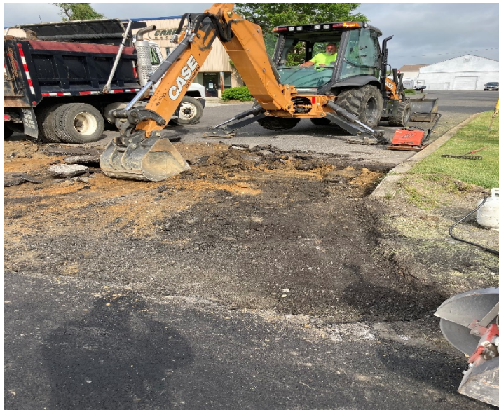
Figure 7: Contractor prepped driveway for Hot Mixed Asphalt.
