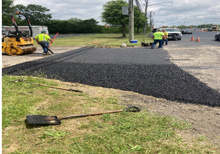
Figure 8: Contractor preparing to roll out driveway.
