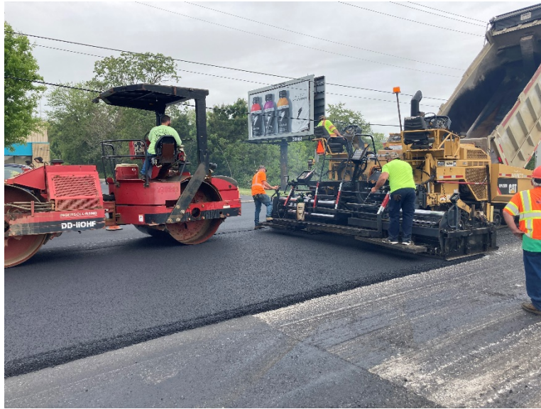
Figure 6: 12.5M HMA intermediate added Northbound sections 155-161.
