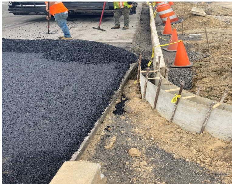
Figure 6: 12.5M HMA intermediate added Northbound sections 155-161.
