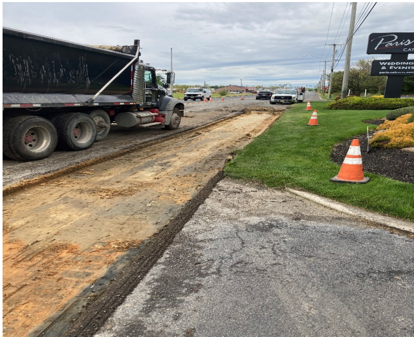
Figure 1: Contractor milling north of New Freedom rd. on Berlin Cross Keys Rd.
