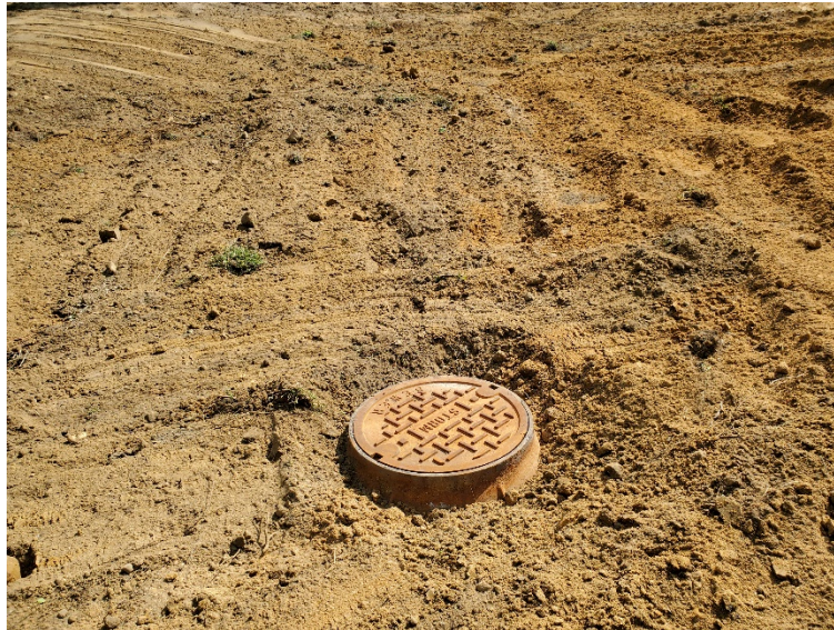
Figure 8 New storm manhole casting after backfilling at Sta. 144+94
