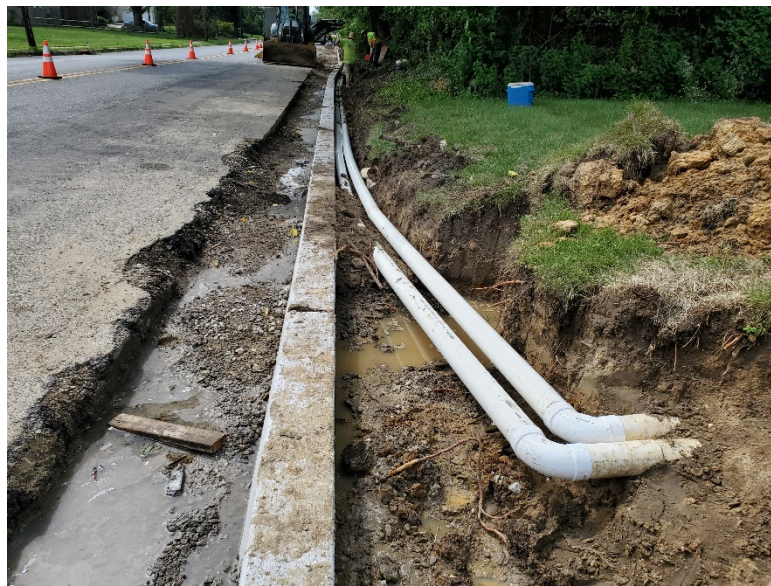
Figure 15 Existing underdrain pipes connected to the inlet sidewall at Sta. 113+39
