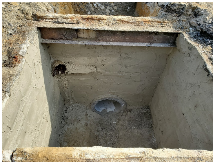
Figure 9 Northern storm drainage inlet at Sta. 144+94 reconstructed with new 15" reinforced concrete pipe connected. 18" reinforced concrete pipe was not used and a field modification was needed. Underdrain shown was not tampered with
