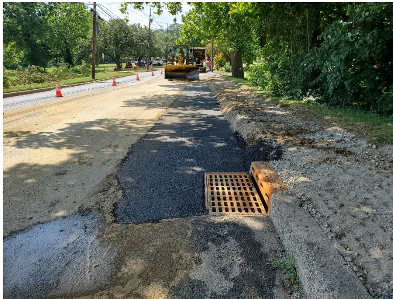
Figure 5 2" HMA applied along WB Kresson road from Sta. 139+73 to Sta. 141+99
