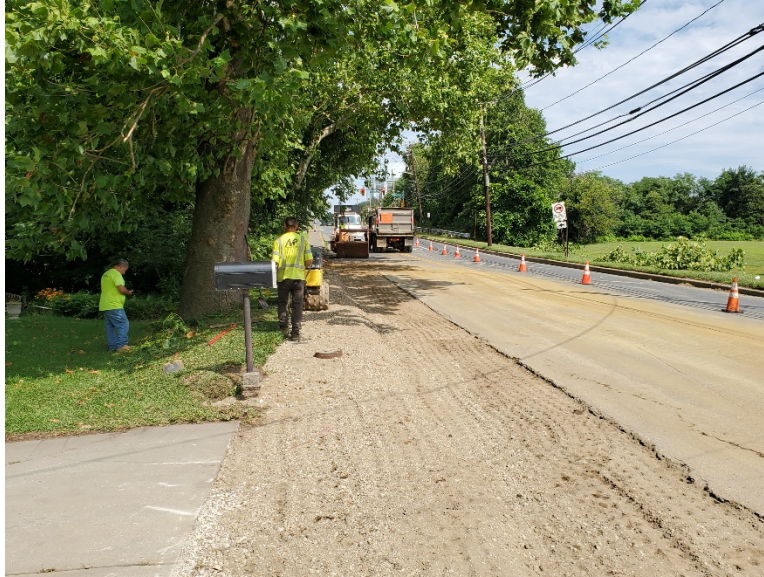
Figure 4 Trench backfilled and compacted along WB Kresson Road
