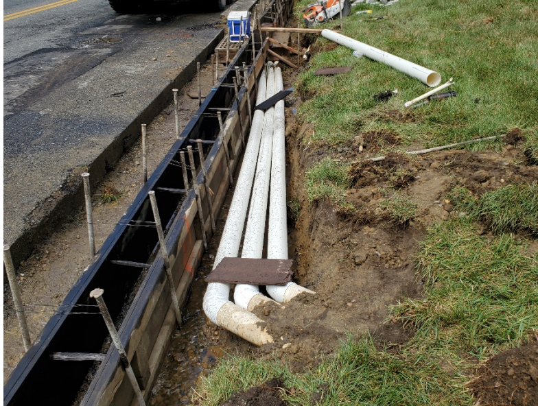
Figure 14 Existing underdrain pipes connected to the inlet sidewall at Sta. 117+03
