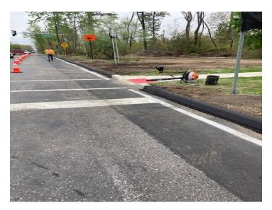
Figure 2 & 3: HMA curb installation Northbound Berlin Cross Keys Rd.
