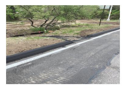
Figure 4&5: HMA curb installed with separation for proper drainage.
