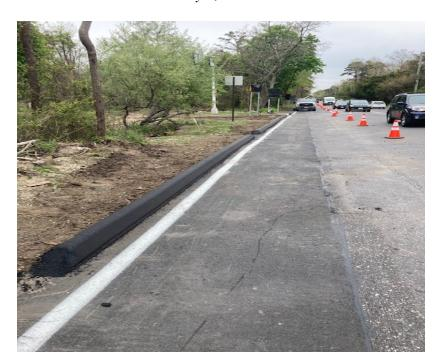
Figure 1: Contractor installed HMA curb Northbound Berlin Cross Keys Rd.
