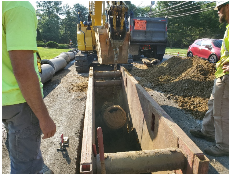
Figure 2 Excavating trench which comprise of removing existing 18" RCP along WB Kresson Road
