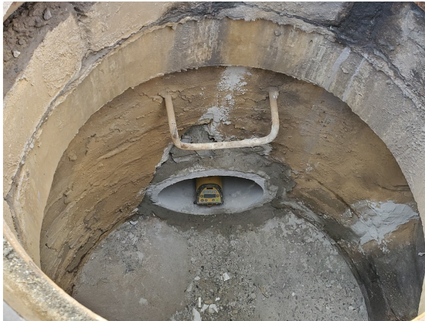
Figure 7 Reconstruction of the storm manhole located at Sta. 121+57 facing East
