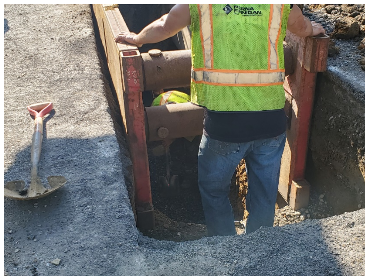
Figure 3 Laborers adjusting DGA bedding for pipe placement. Laser system being used to align RCP to proper elevation. The trench box was used on trench depths of 5ft or more
