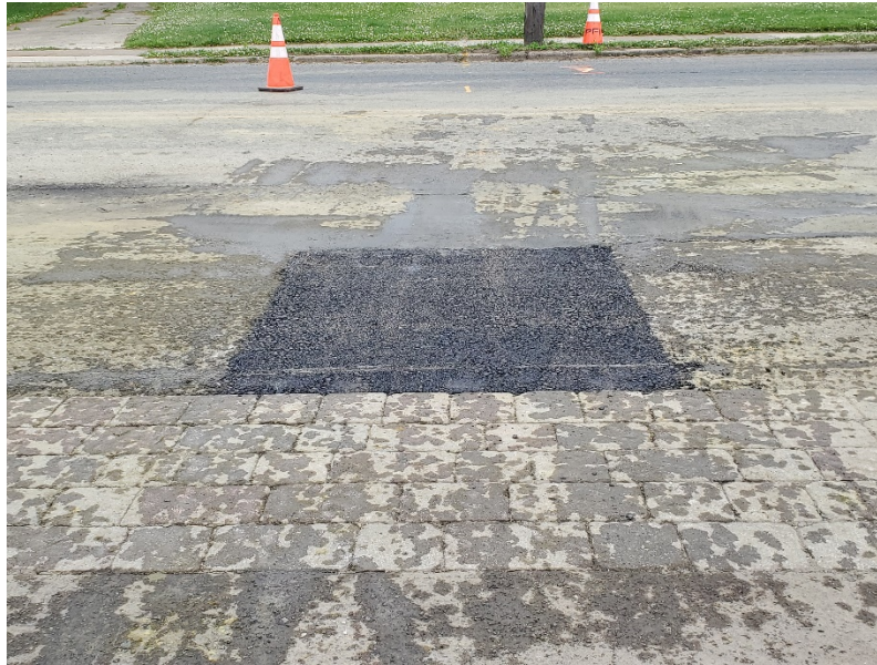
Figure 12 Trench used by PSEG was backfilled. 8" HMA used by contractor to properly meet existing roadway
