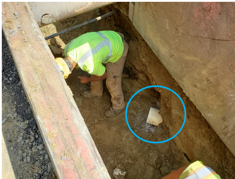
Figure 13 An 8" PVC sanitary line was impacted during removal of existing storm drainage pipe
