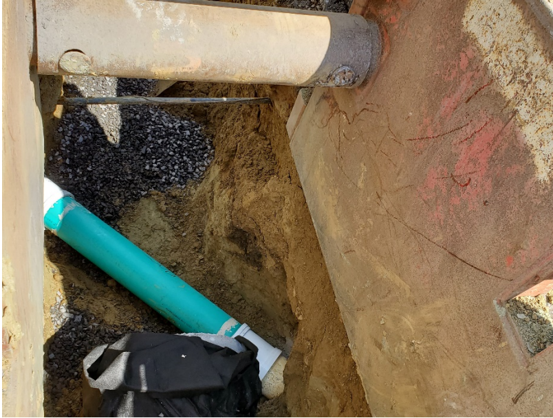
Figure 14 Contractor connected new 8" PVC to the existing pipe using sleeves
