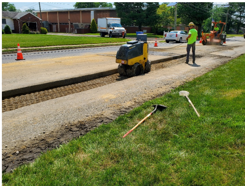
Figure 14 Vibrating trans compactor used to compact backfill before HMA application
