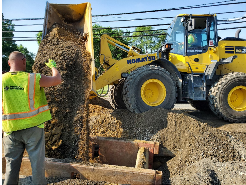
Figure 6 Backfill placed after RCP is installed
