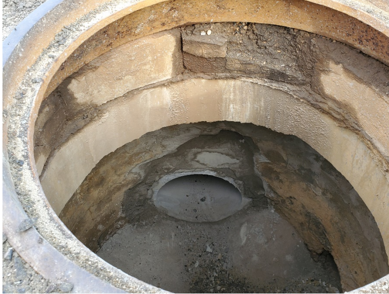
Figure 8 Reconstruction of the storm manhole located at Sta. 121+57 facing West
