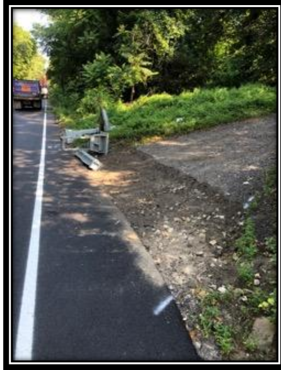
Figure: 2 – Preparation of subbase before installation of HMA driveway along the northbound lane between Carriage Stop Drive and Berlin-Clementon Road in the Borough of Berlin
