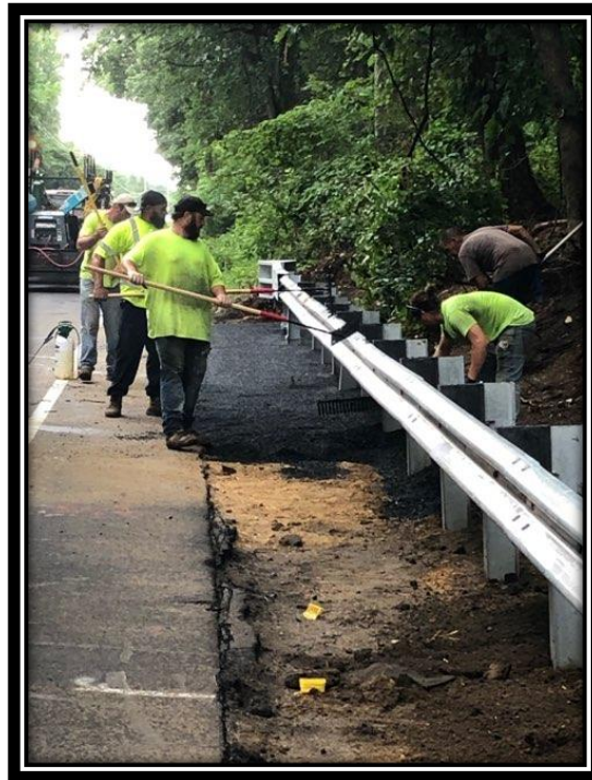
Figure: 3 – Installation of HMA non vegetative surface under the newly installed beam guide rail along the southbound lane between Berlin-Clementon Road and Carriage Stop Drive in the Borough of Pine Hill
