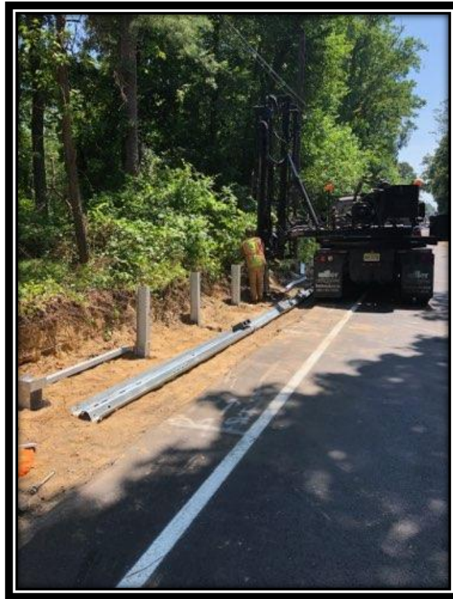
Figure: 1 – Installation of beam guide rail along the southbound lane between Berlin-Clementon Road and Carriage Stop Drive in the Borough of Pine Hill
