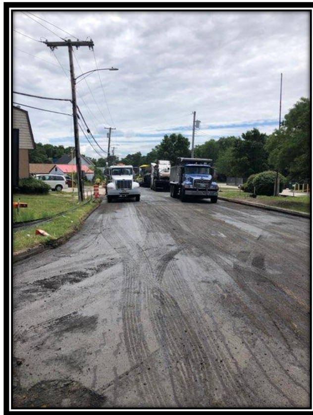
Figure: 1 – Installation of HMA 19M64 base course in the northbound lane between Smith Terrace and the White Horse Pike in the Borough of Clementon
