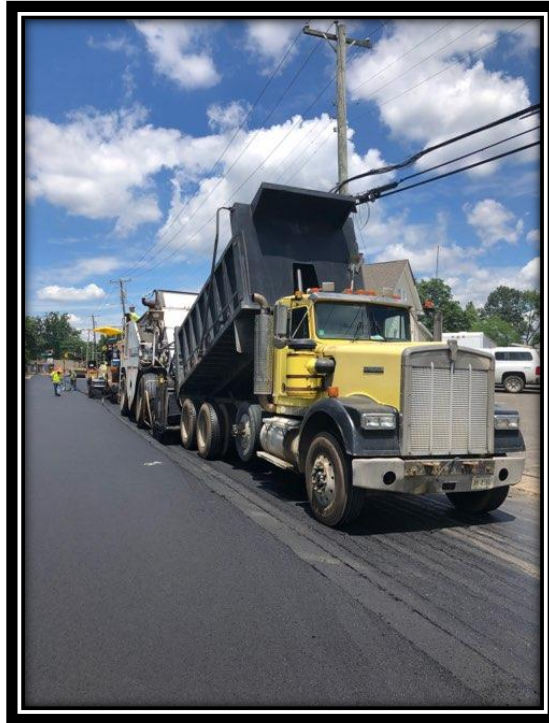
Figure: 2 – Installation of HMA 9.5M64 surface course in the southbound lane between the White Horse Pike and Berlin-Clementon Road in the Borough of Clementon
