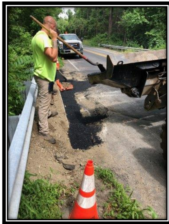
Figure: 3 – Road restoration at the newly installed storm sewer improvements along the southbound lane between Berlin-Clementon Road and Berlin-Cross Keys Road in the Borough of Pine Hill
