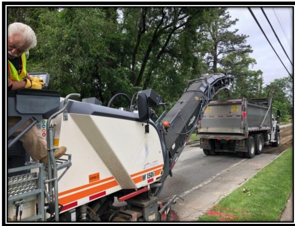
Figure: 2 – Removal of existing asphalt along gutters prior to full depth reclamation with cement between the White Horse Pike and Berlin Clementon Road in the Borough of Clementon
