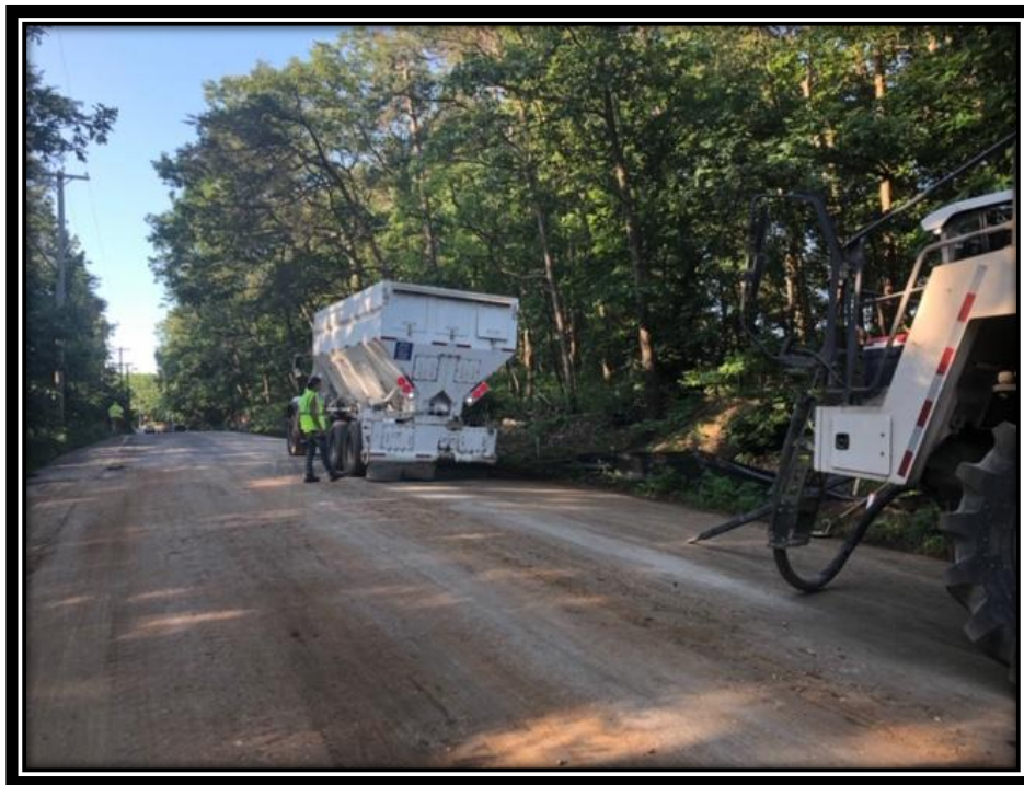
Figure: 3 – Full depth reclamation with cement between the White Horse Pike and Berlin Clementon Road in the Borough of Clementon
