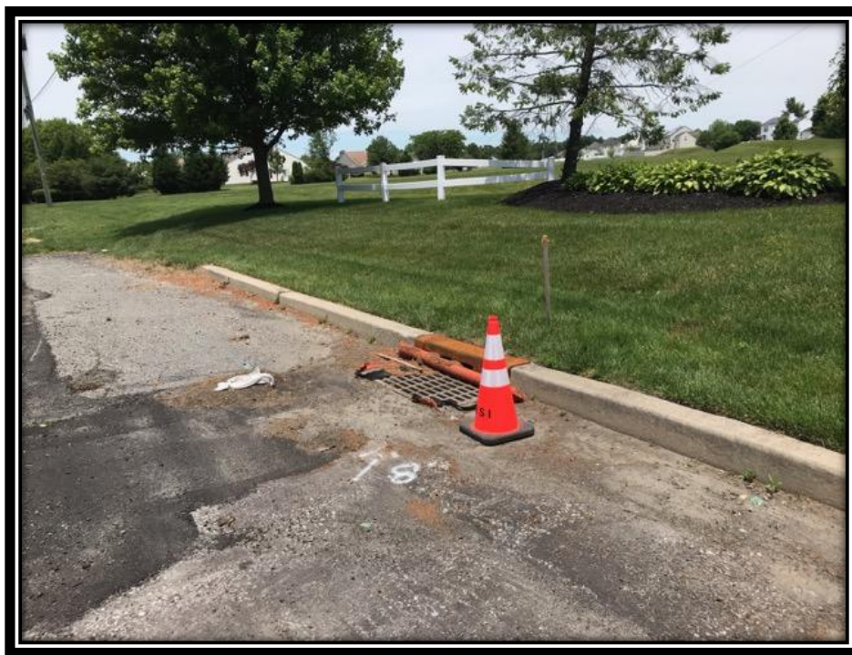
Figure: 3 – Installation of type 'N' eco inlet curb piece along the northbound lane between Westbury Drive and Carriage Stop Drive in the Borough of Berlin
