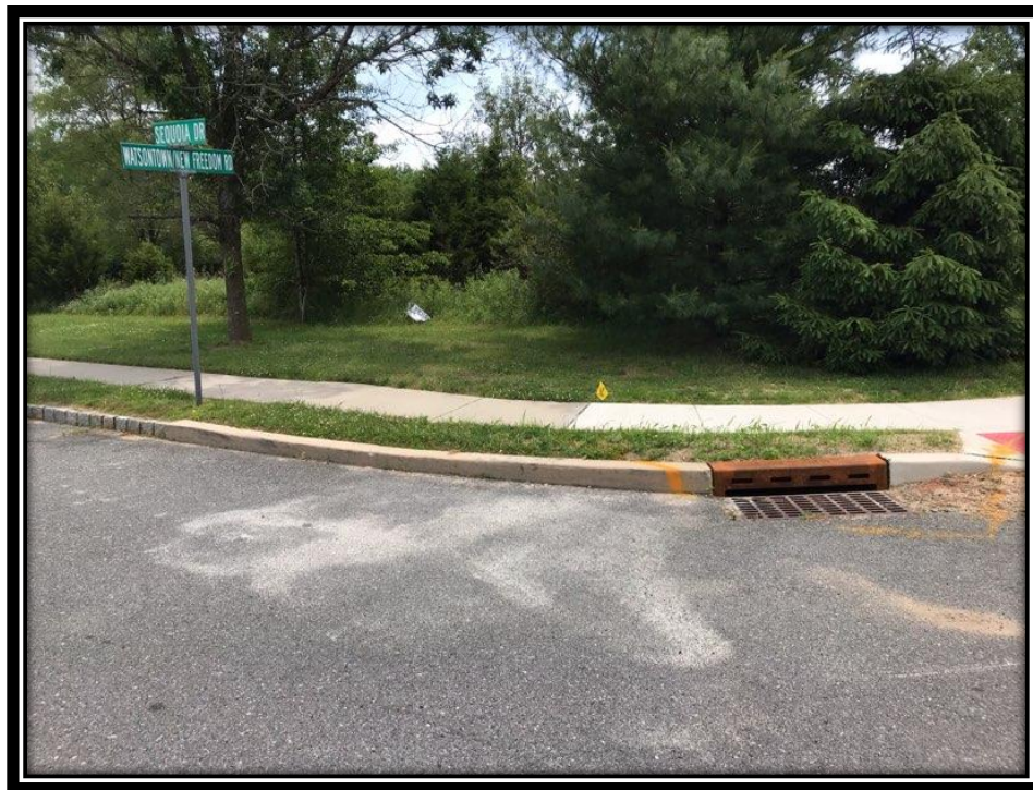
Figure: 2 – Installation of type 'N' eco inlet curb piece along the northbound lane at the intersection with Sequoia Drive in the Borough of Berlin
