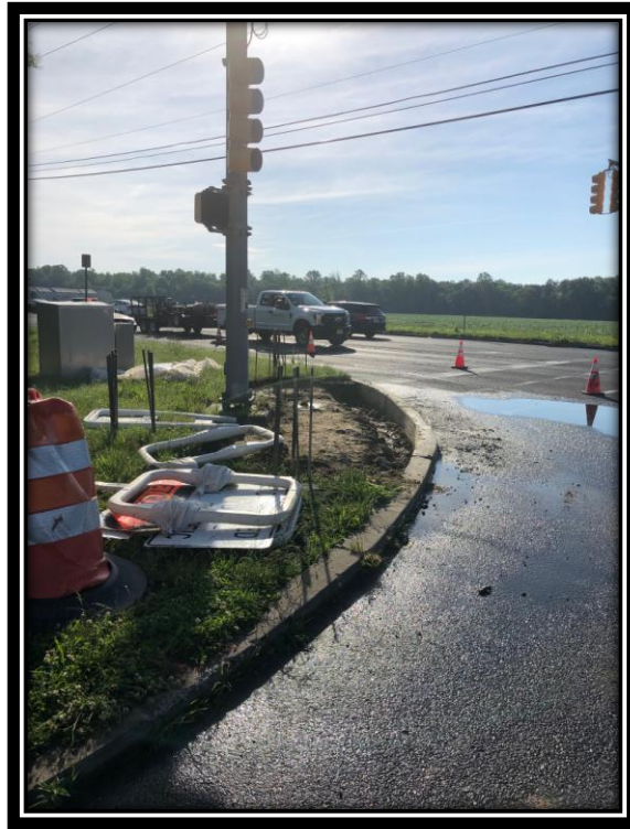
Figure: 2 – Installation of concrete curb for the proposed ADA ramp at the northeast corner of the intersection with Berlin-Cross Keys Road in the Borough of Berlin
