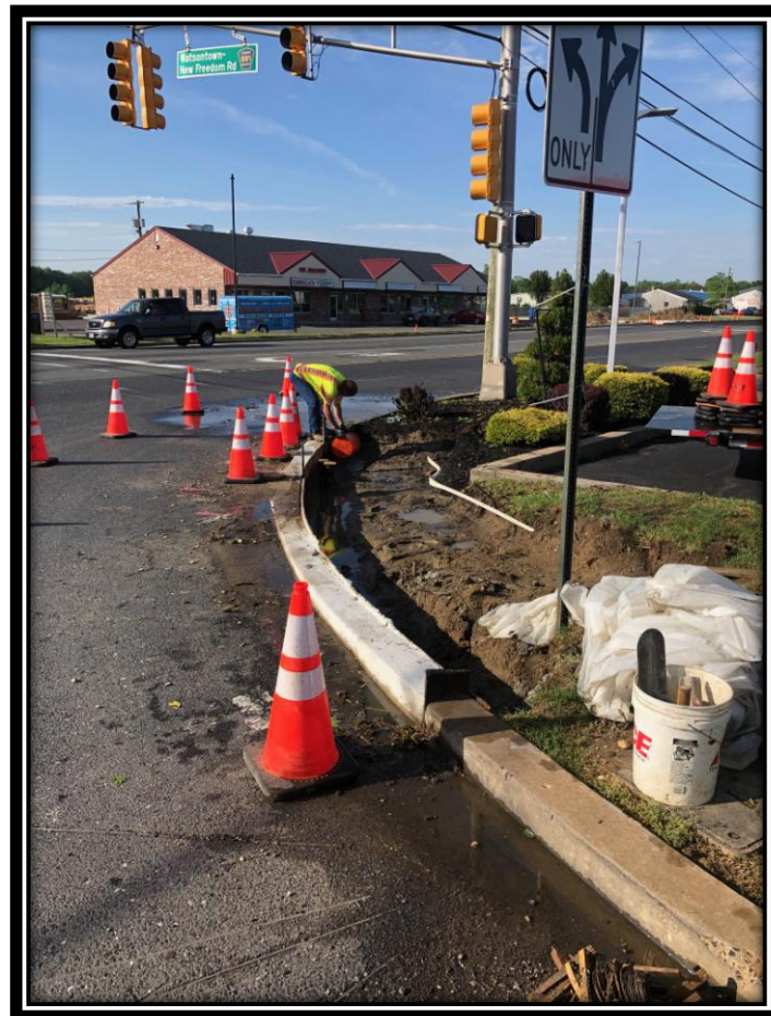
Figure: 1 – Installation of concrete curb for the proposed ADA ramp at the northwest corner of the intersection with Berlin-Cross Keys Road in the Borough of Berlin
