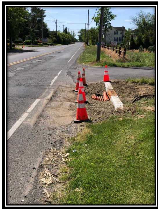
Figure: 3 – Installation of concrete curb along the southbound lane between Carriage Stop Drive and Westbury Drive in the Borough of Pine Hill
