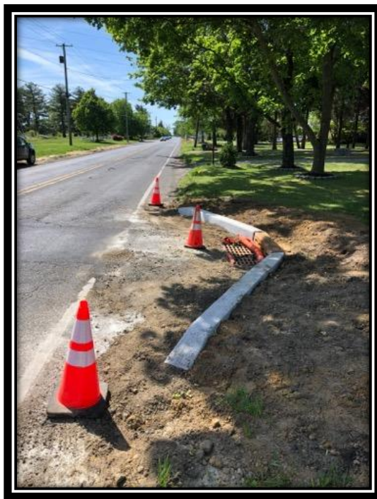
Figure: 3 – Installation of concrete curb along the northbound lane between Wyndam Road and Westbury Drive in the Borough of Berlin
