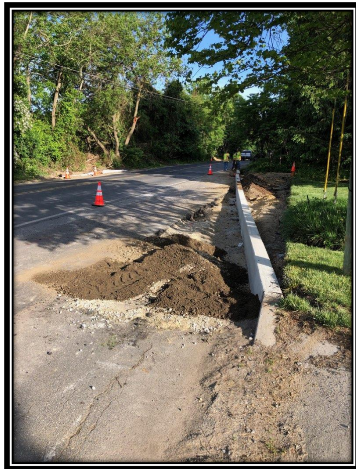
Figure: 1 – Installation of concrete curb in the northbound acceleration lane just past the intersection with Carriage Stop Drive in the Borough of Berlin
