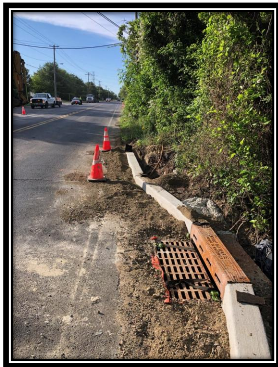
Figure: 2 – Installation of concrete curb along the southbound lane between Berlin-Clementon Road and Carriage Stop Drive in the Borough of Pine Hill
