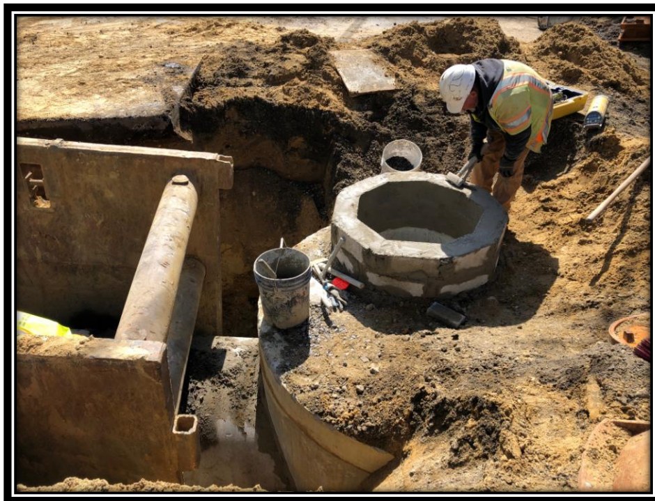
Figure: 2 – Installation of a 6' diameter storm manhole in the southbound lane of Watsontown-New Freedom Road (CR 691) in the Borough of Pine Hill
