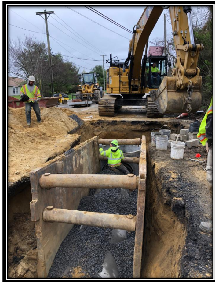
Figure: 1 – Installation of 36" RCP along the southbound lane of Watson-town-New Freedom Road (CR 691) in the Borough of Pine Hill
