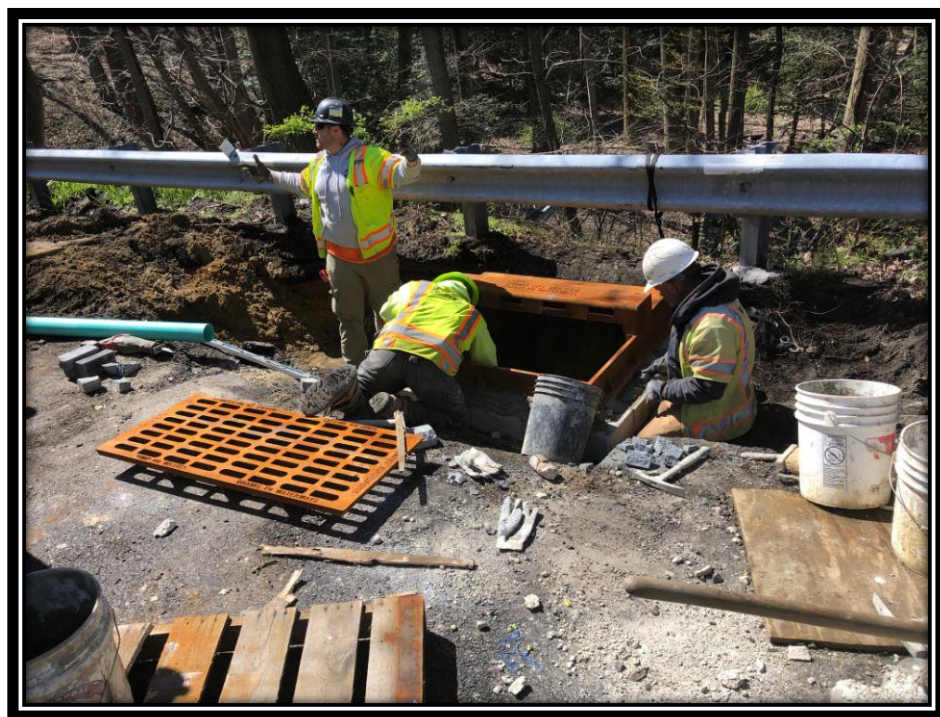
Figure: 3 – Installation of type 'B' inlet in the southbound lane of Watsontown-New Freedom Road (CR 691) in the Borough of Pine Hill
