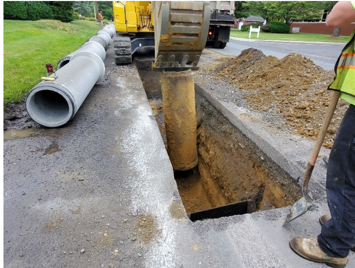
Figure 2 Excavating trench which comprise of existing 18" RCP removal along WB Kresson Road
