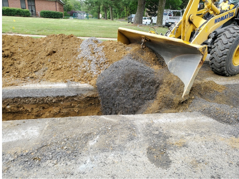
Figure 6 Backfill placed after RCP is installed
