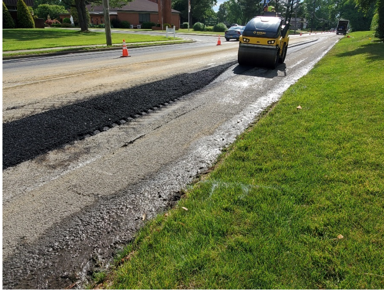
Figure 14 Rolling compactor used to compact and even out the 8" HMA to meet existing roadway
