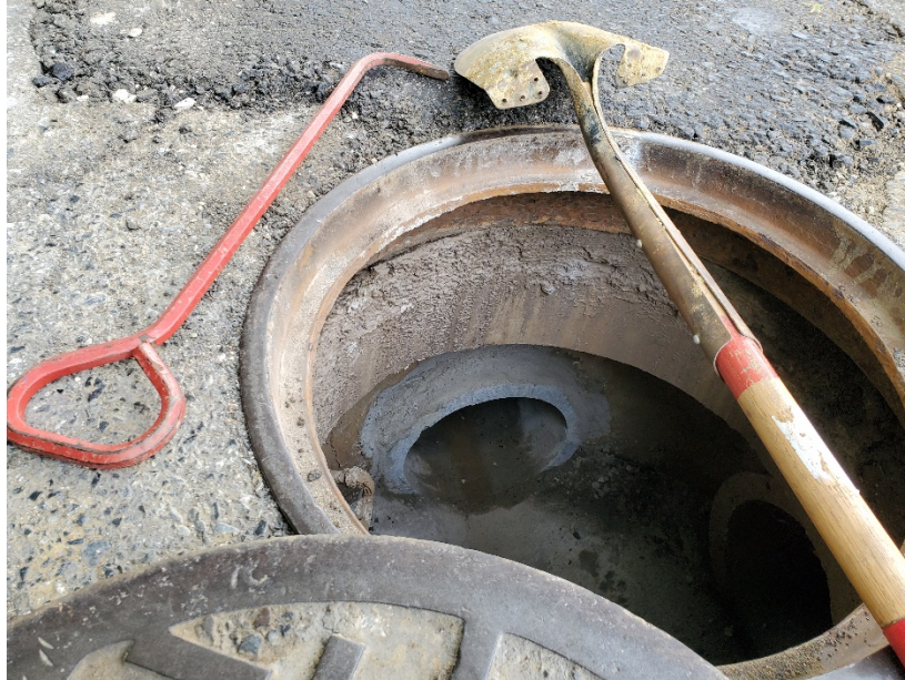
Figure 10 Reconstruction of the storm manhole located at Sta.113+55
