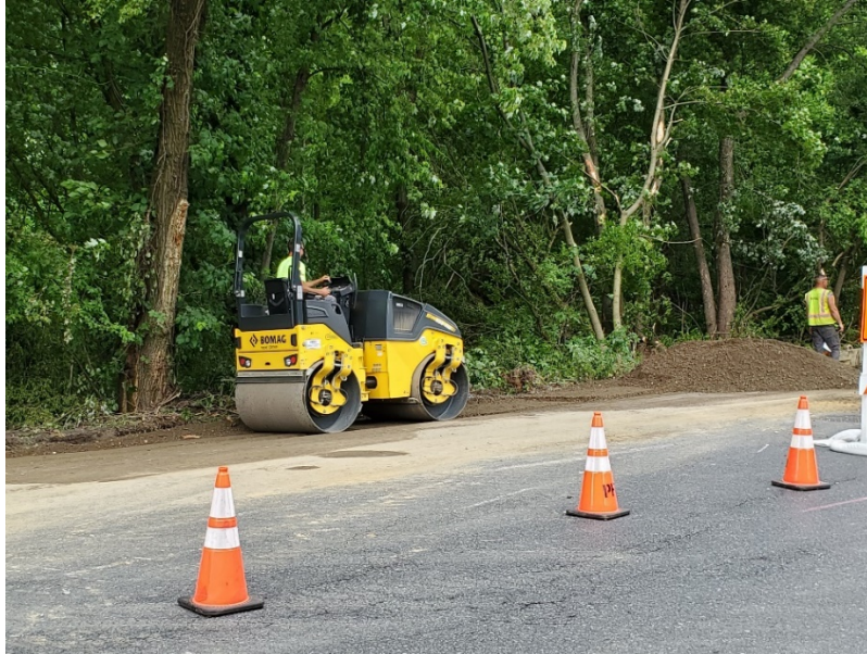
Figure 12 Rolling compactor used to level backfill at the end of the day
