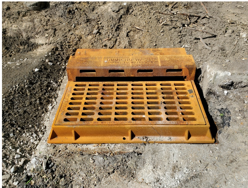
Figure 9 New casting for the storm drainage inlet located at Sta. 113+40
