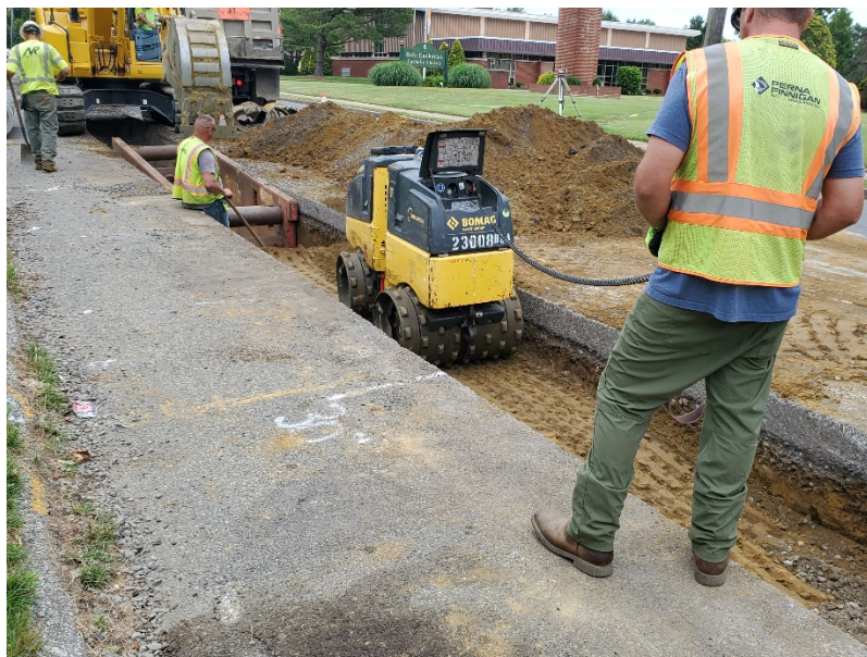
Figure 13 Vibrating trans compactor used to compact backfill before HMA application
