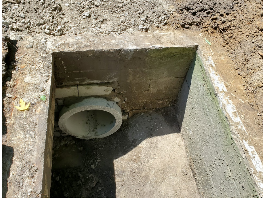
Figure 8 Reconstruction of the storm drainage inlet located at Sta. 113+40
