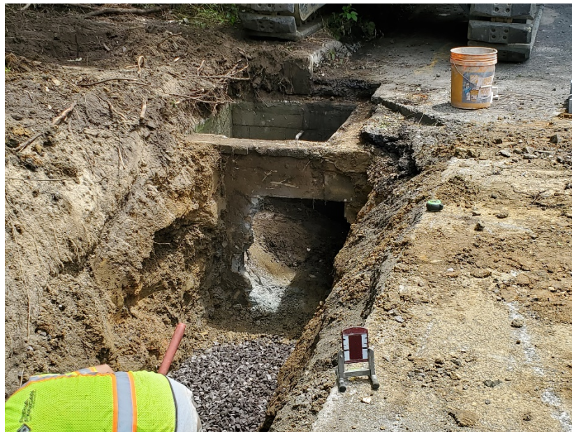
Figure 7 Existing storm drainage inlet located at Sta. 113+40 being demolished
